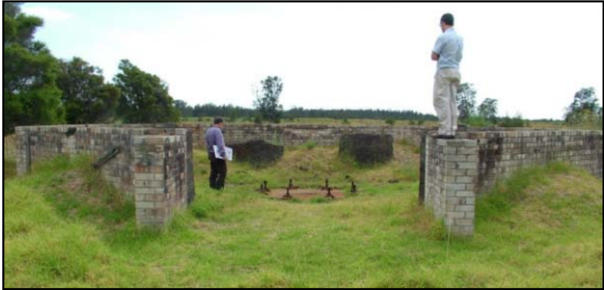
Looking towards the north western former WWII gun emplacement.
