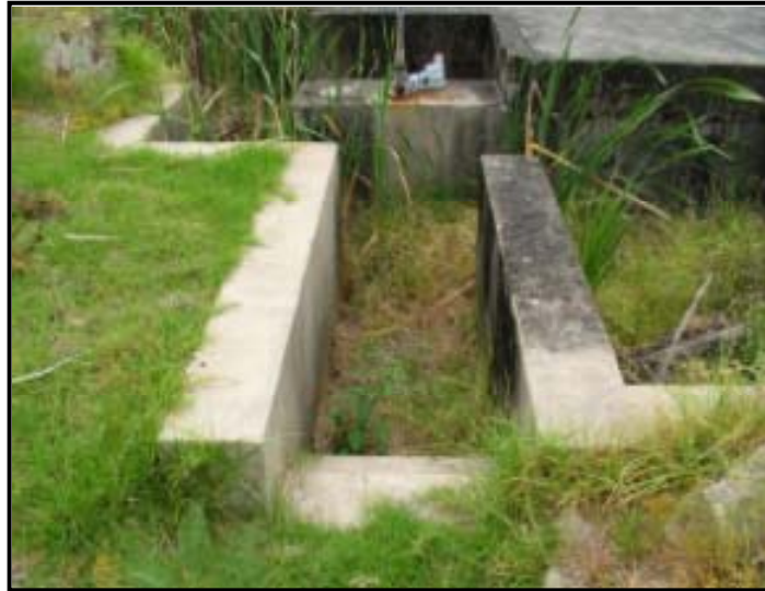
Looking towards the stairway entry into the WWII underground command post.
