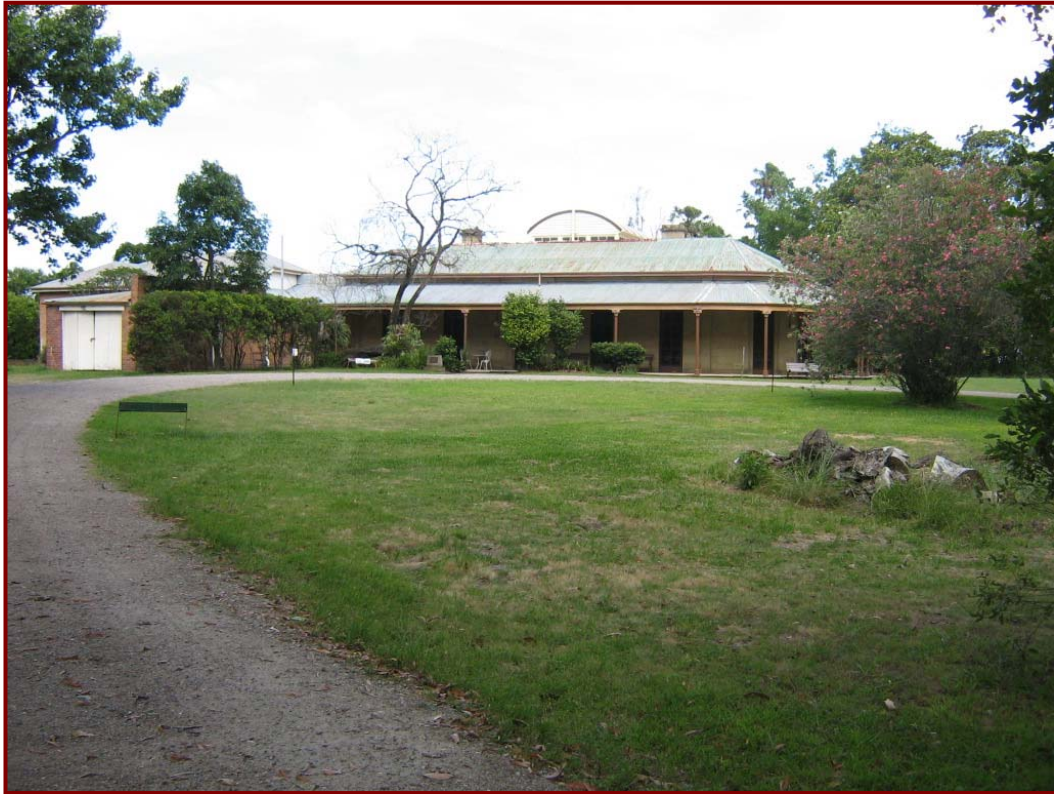
Tomago House adjoining to the North of the subject site.
