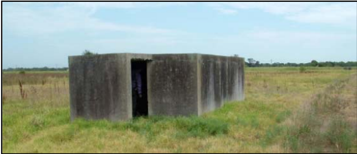
Looking towards a WWII ammunition bunker on the site.
