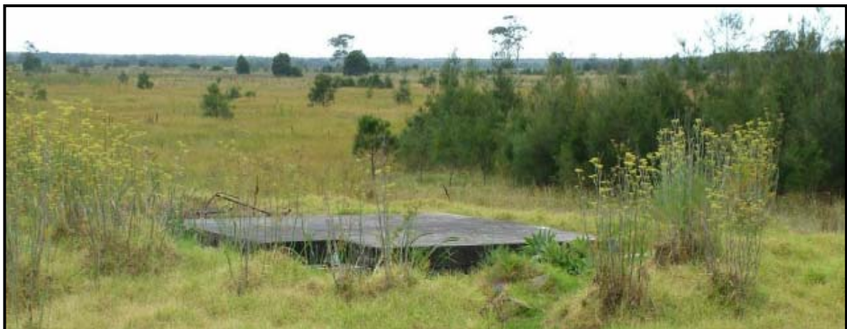
Looking towards the WWII underground command post.
