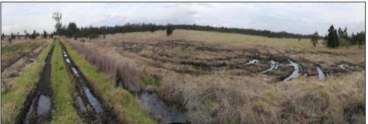
Figure 3 - Saturated ground surface along access track and adjacent paddock
