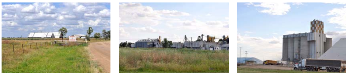
Plate 5. Typical photos toward agricultural and industrial structures
