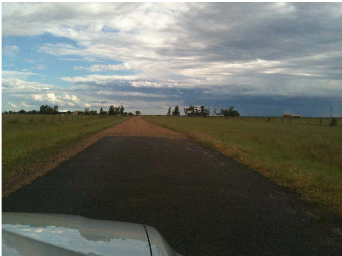
Barton Plains Road southbound at end of bitumen seal
