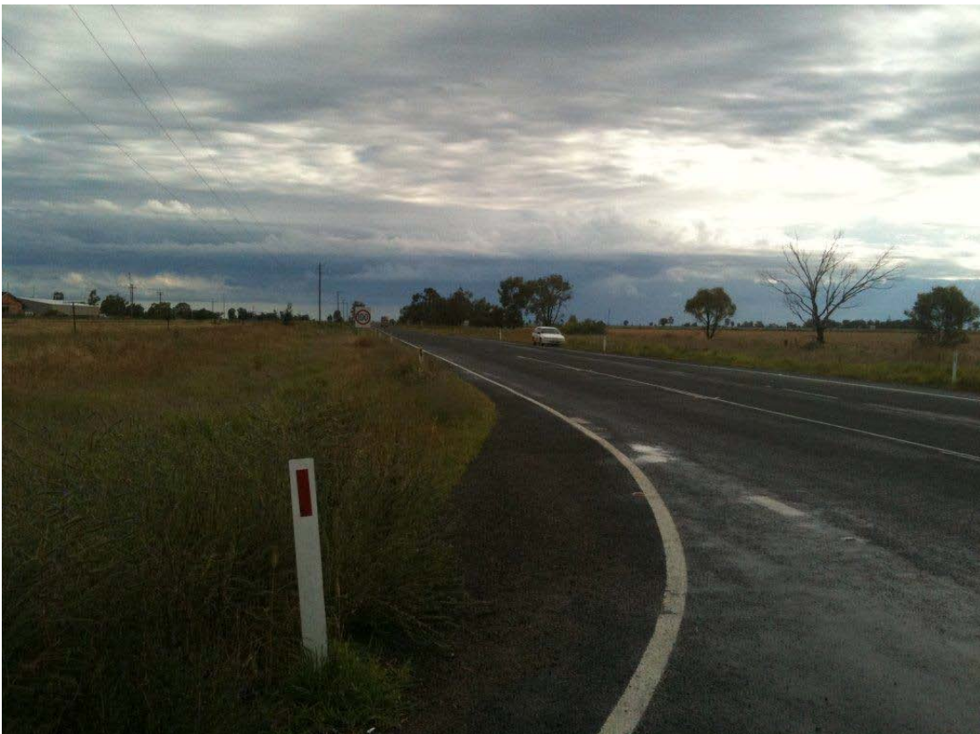
Newell Highway southern approach to Burrington Road
