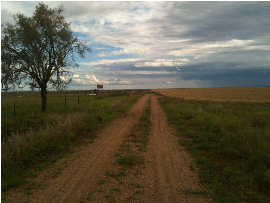
Barton Plains Road at site
