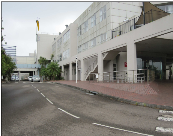
Figure 5: Former Hospital Entrance
