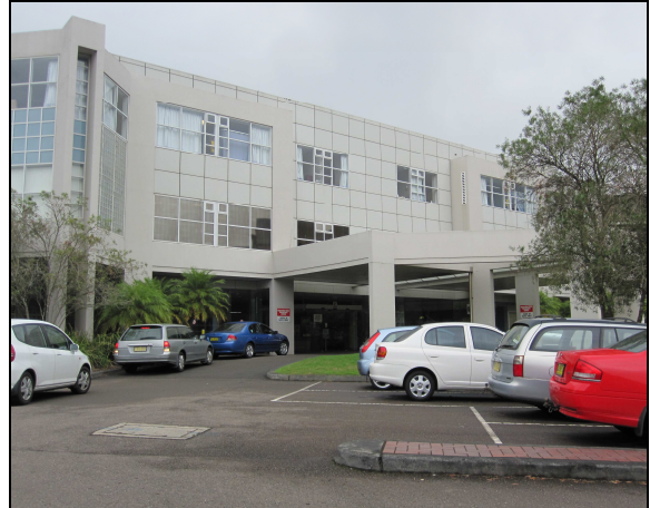
Figure 3: Former Hospital Entrance
