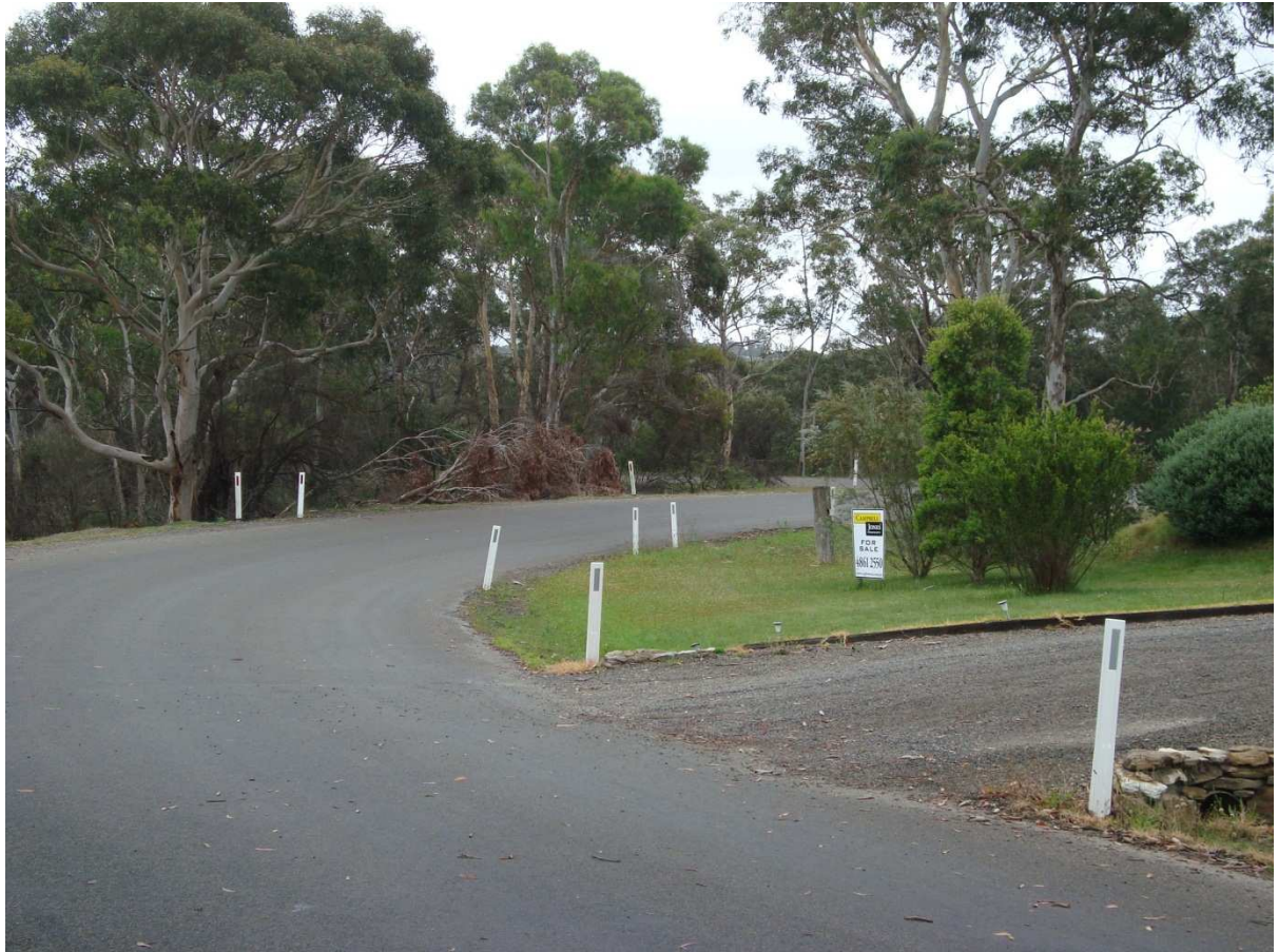
Medway Rd....narrow, limited line of sight, driveway
