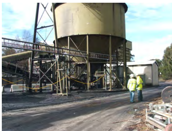
(b) Coal ROM bin (450 t)
