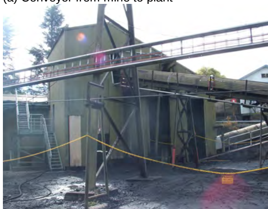
(c) Primary crusher and screen
