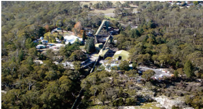
Viewpoint 3 - Looking south east along conveyor
