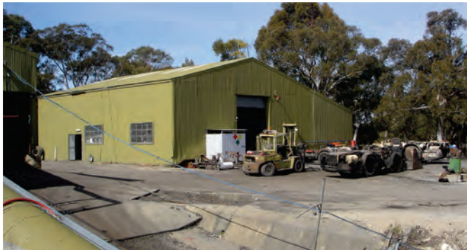
Viewpoint 4 - Looking south towards workshop
