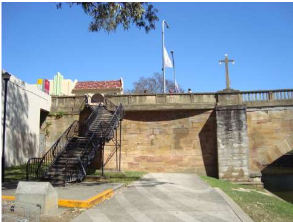
Figure 5: Stairs from Parramatta River frontage to Church Street
