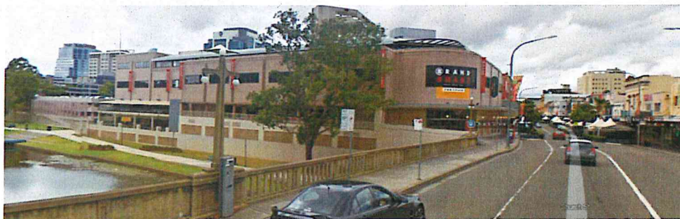
Subject Site as Viewed from the Lennox Bridge
