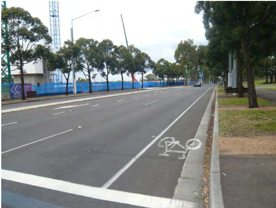
View looking south at the intersection of Australia Avenue with Herb Elliott Avenue.
