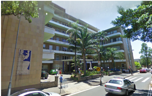
06 BUILDING 13 - KING GEORGE V
