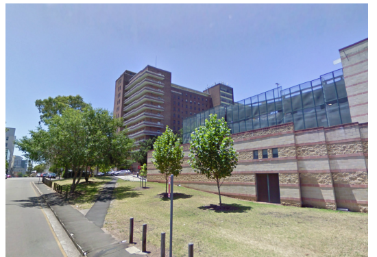
16 QUEEN MARY BUILDING & STAFF CARPARK
