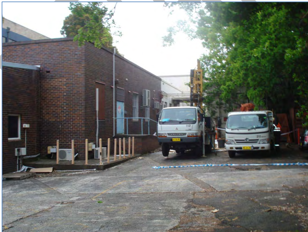
Plate P3: Building 21 from car park.
