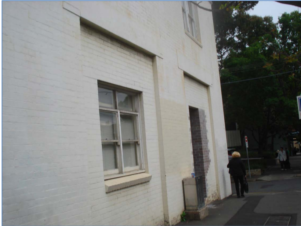
Plate P2: Building 11 from Missenden Road. Previous garage doors are visible, that have been converted to walls and windows.
