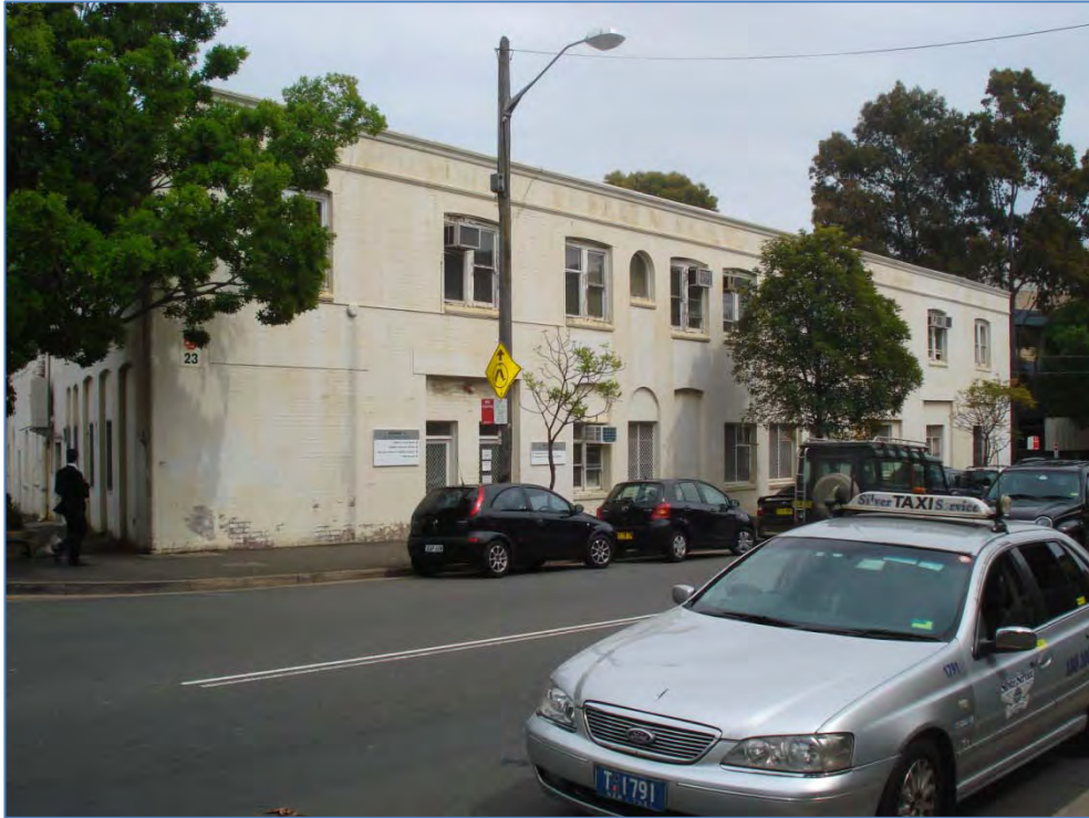
Plate P1: Building 11 from Missenden Road. 'Breville' Signage visible near building roofline.
