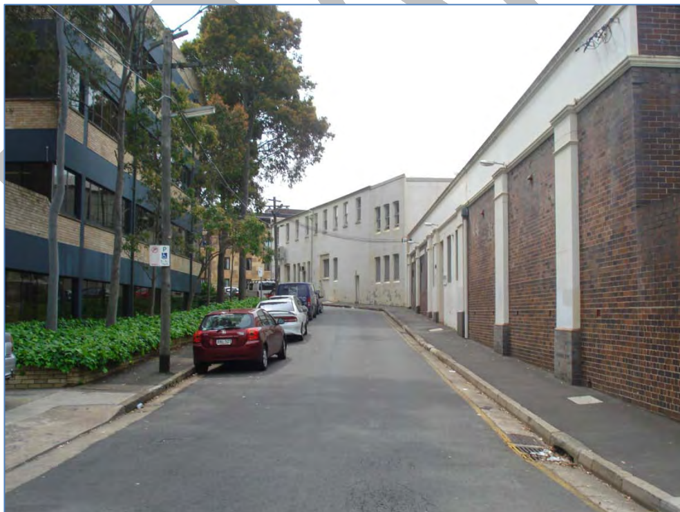
Plate P5: Oxygen tank in car park at rear of Building 21 (foreground right) and Building 11 (background right) viewed from Lucas Street
