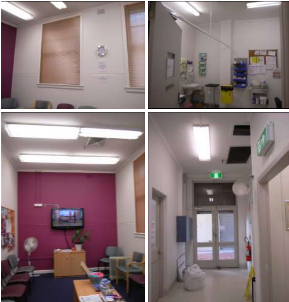
Figure 7: General internal views of Building 21 currently used as RPA Sexual Health services
