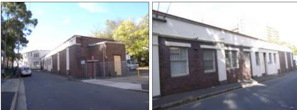
Figure 8: External views of Building 21 along Lucas Street
