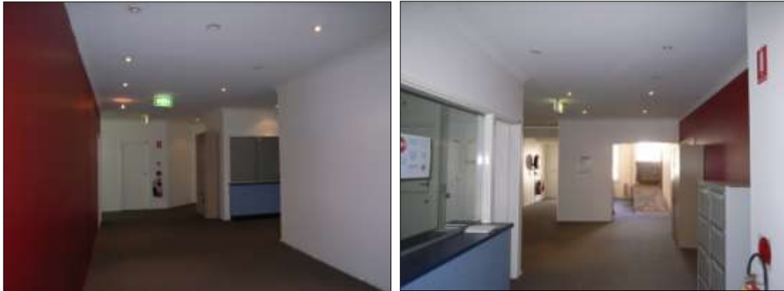
Figure 4: Internal configuration and finishes of the upper floor of Building 11
