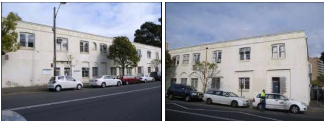
Figure 5: Missenden Road elevation of Building 11 with bricked in former loading docks and modified openings. This section of the building is outside of the development site
