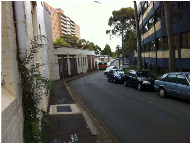
Fig 1 Existing LV overhead supply to site
