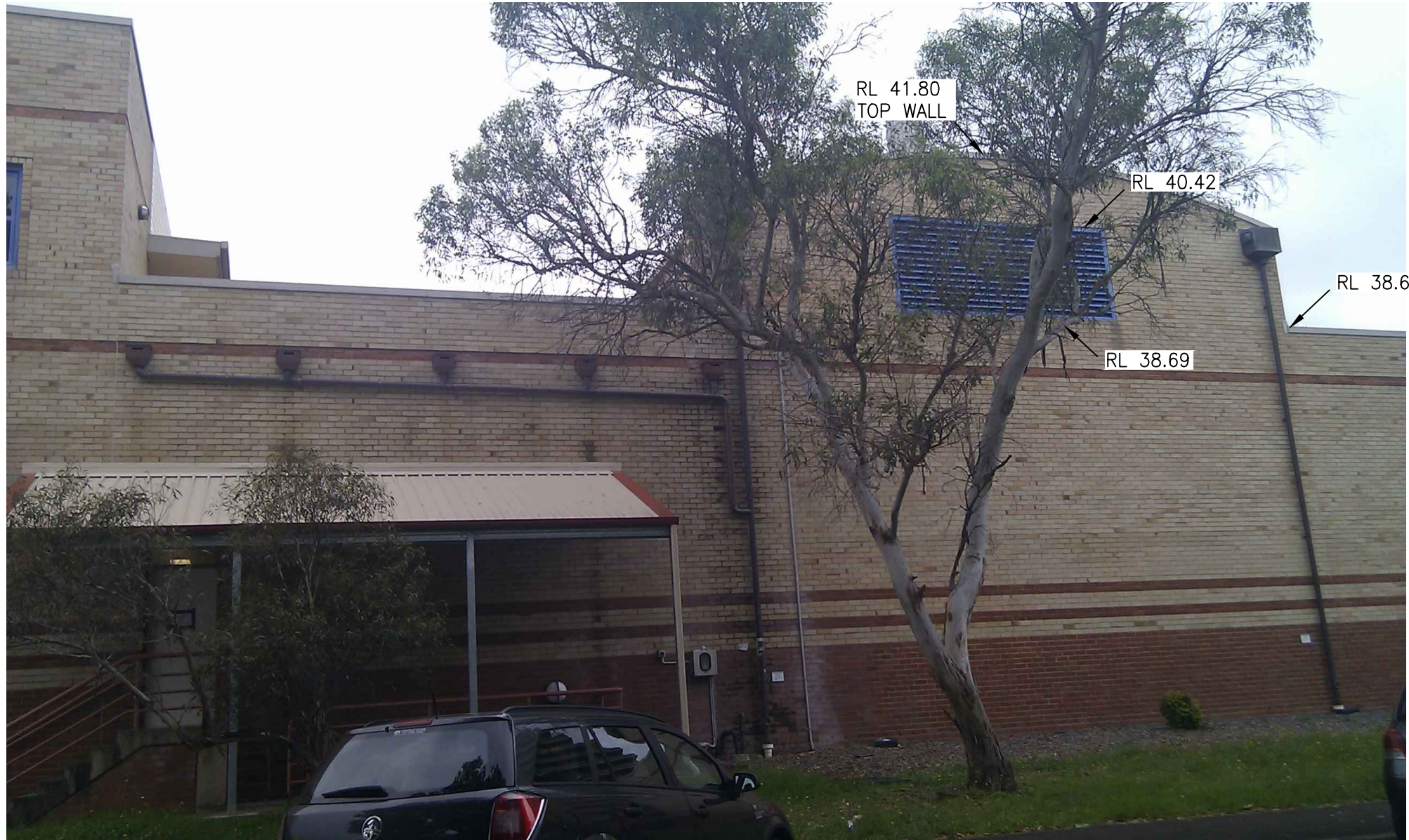
PHOTO # 2 "CYCLOTRON BUILDING"
