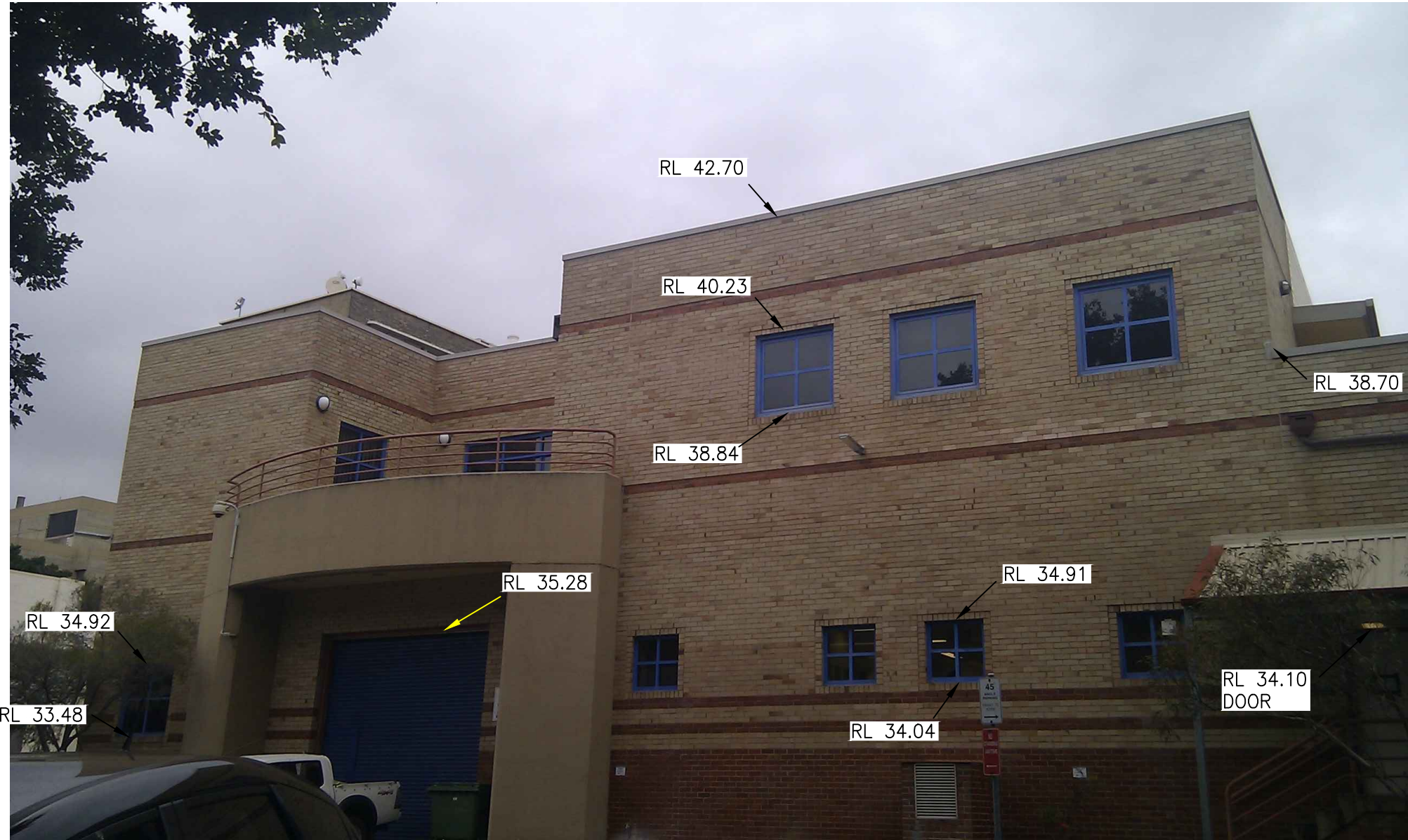
PHOTO # 1 "CYCLOTRON BUILDING"
