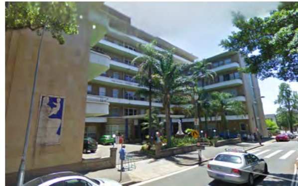
06 BUILDING 13 - KING GEORGE V
