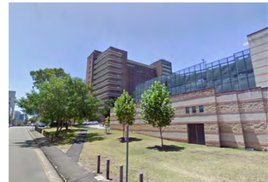
16 QUEEN MARY BUILDING & STAFF CARPARK
