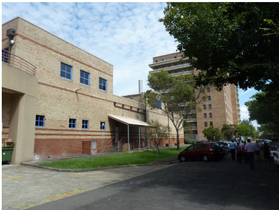
Figure 9 – Cyclotron building to the south of the site with Queen Mary Building in background
