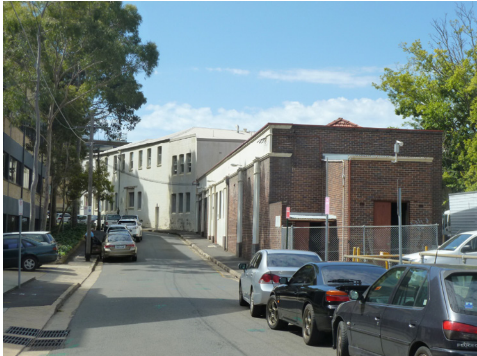
Figure 7 – Building 21 and Building 11 fronting Lucas Street
