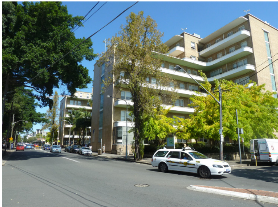
Figure 14 – King George V Building fronting Missenden Road
