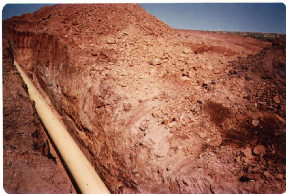
Trench through old levee sediments at site BY/6
