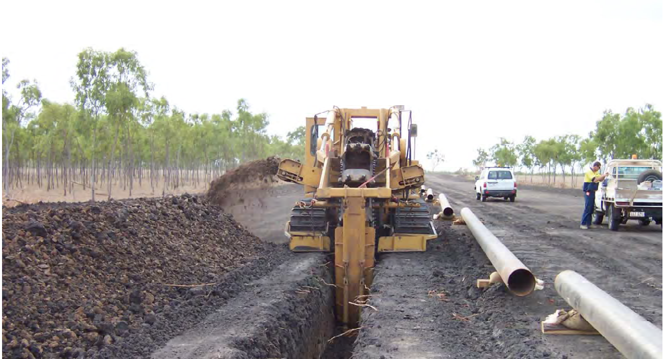
Figure 3 – Typical trenching methods would be used for the majority of the route
