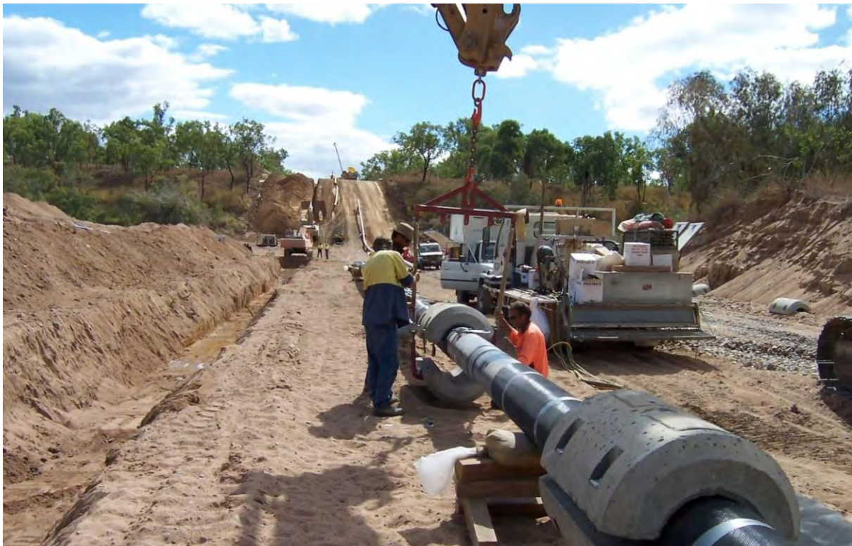
Figure 5 – Adding concrete weights at a watercourse crossing
