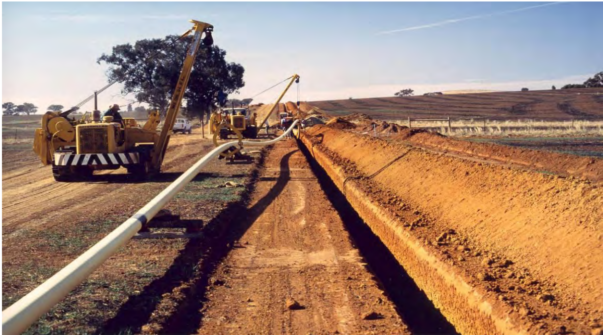
Figure 4 – Typical lowering activity methods would be used for the majority of the route
