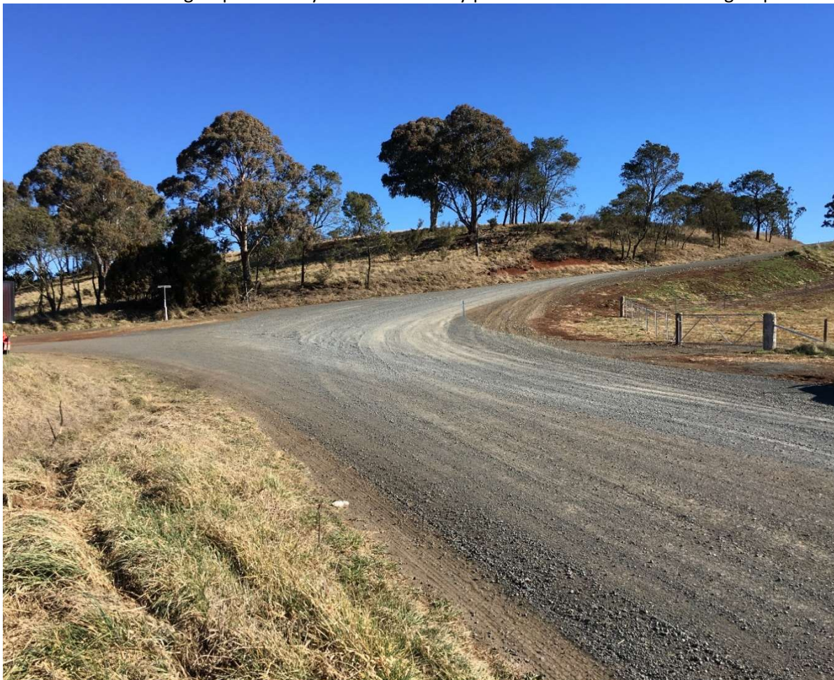
Plate 6.19 Intersection of Maybole and Kelleys Road – Upgraded as part of Stage 1 for OD transport
