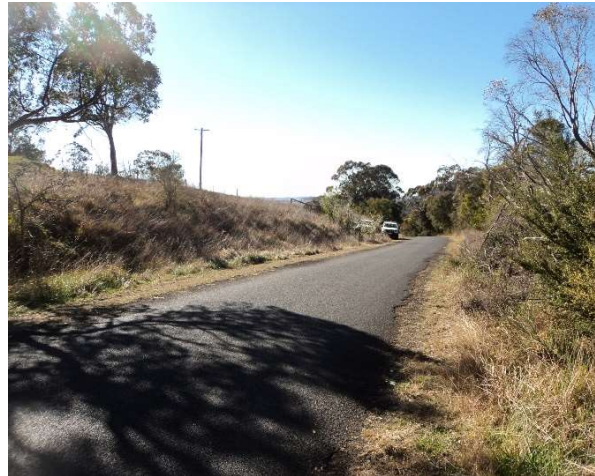
Plate 6.18 View to east on Maybole Road to entry point to southeastern turbine group
