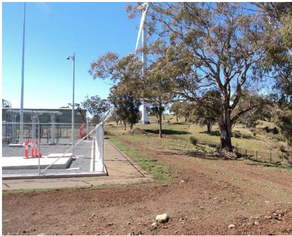
Plate 2.2 Access past Stage 1 substation
