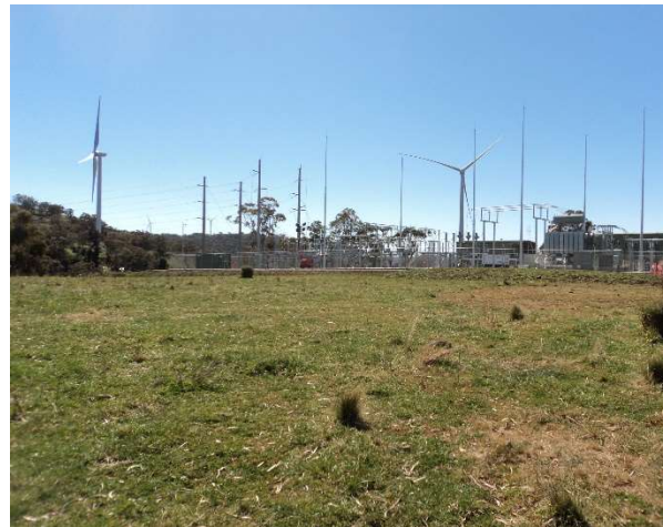
Plate 2.3 Area for extension of substation
