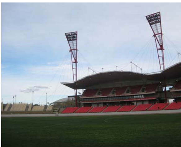
Picture 5 – Existing stands and lighting towers
