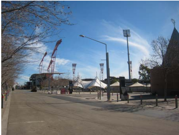
Picture 1 – The Showground Main Arena viewed from Grand Parade looking west
