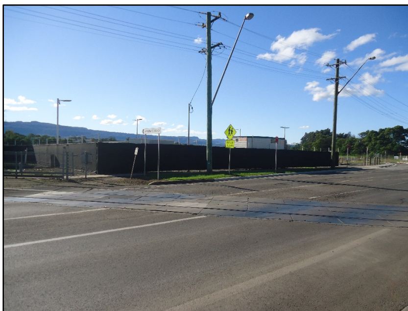
Plate 2: View of location of proposed relocated Gas Pressure Reduction facility from Bolong Road.
