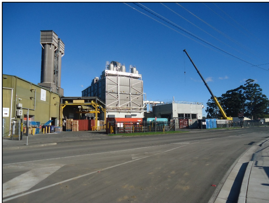
Plate 3: View of Packing Plant, Starch Dryer No. 5 building, and specialty Product Building under construction opposite location of GPRS.
