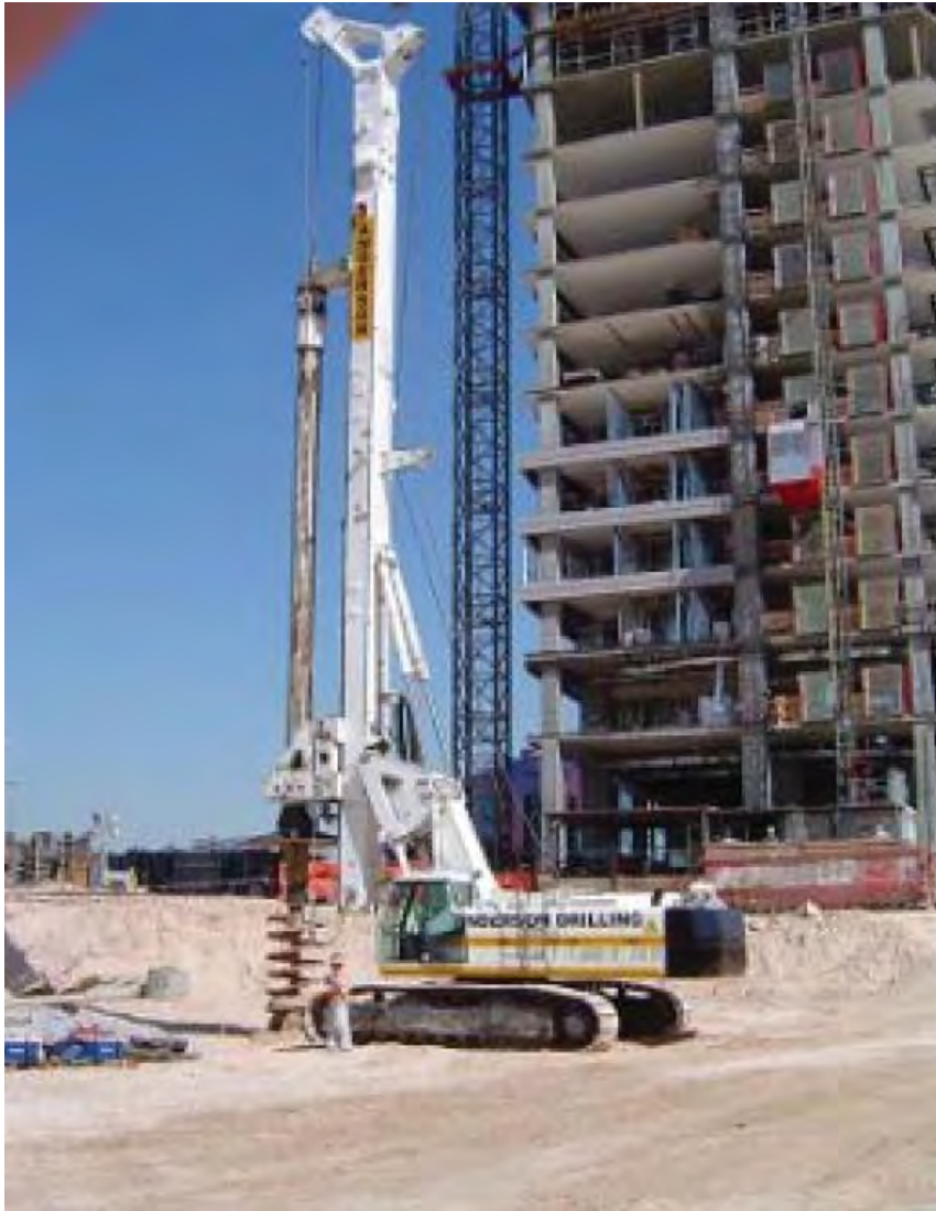
Figure 9-1 Piling rig
