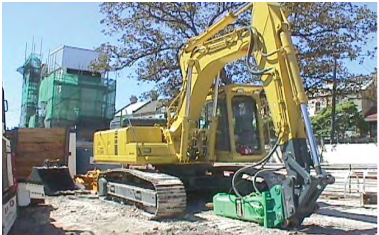
Figure 9-2 Hydraulic rock breaker
