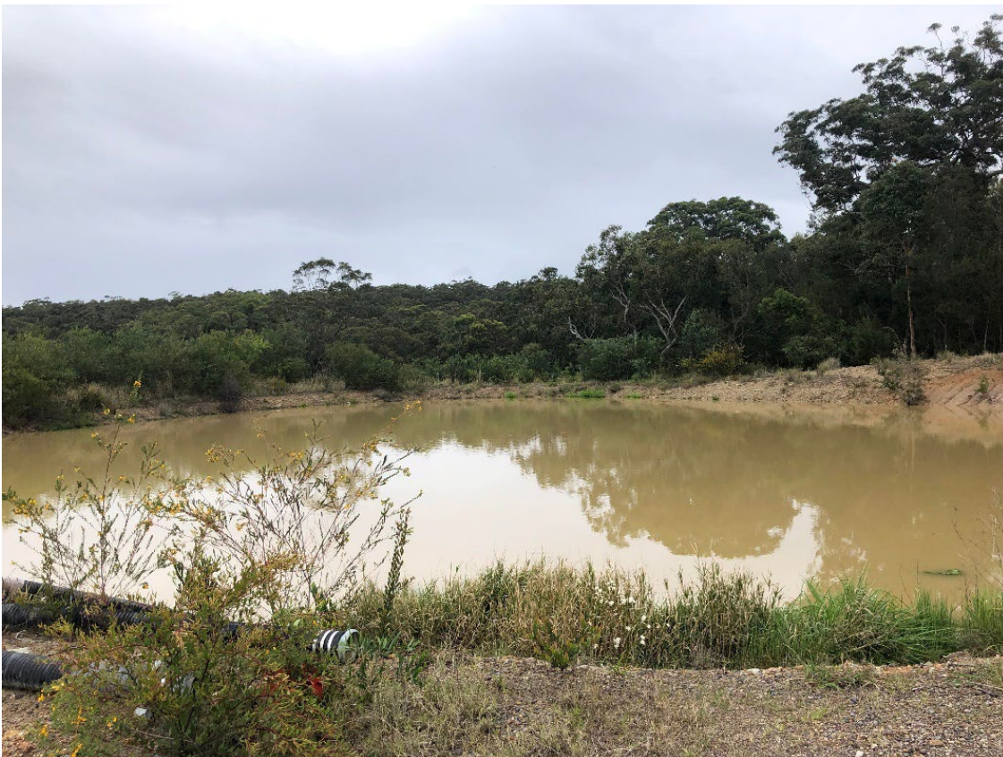
Photograph 6 – Overview of sediment dam
