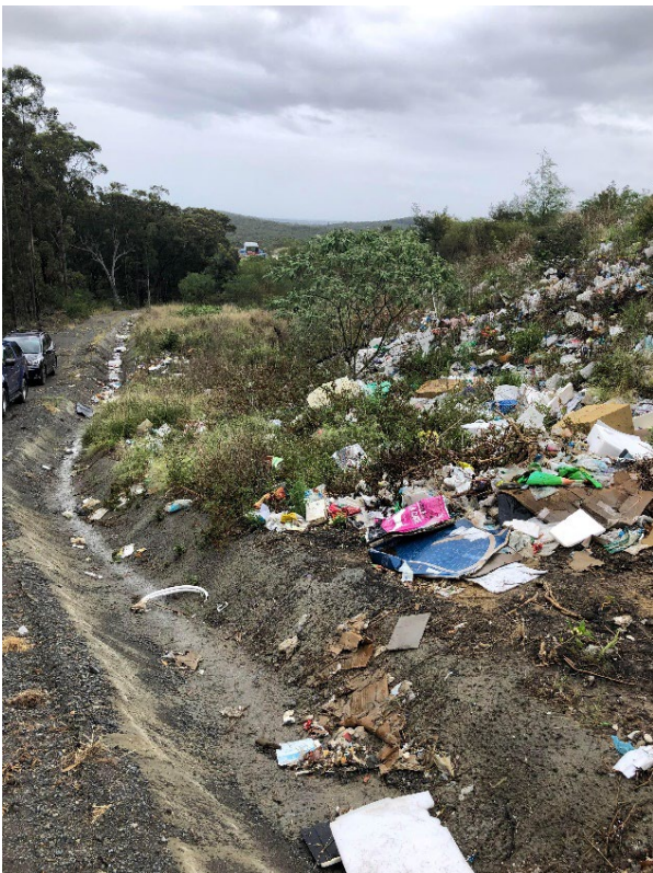
Plate 8 – Stormwater drains filled with litter
