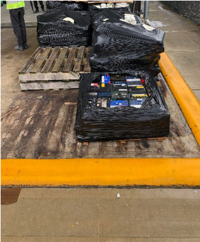
Photograph 11 – Bunding of waste batteries
