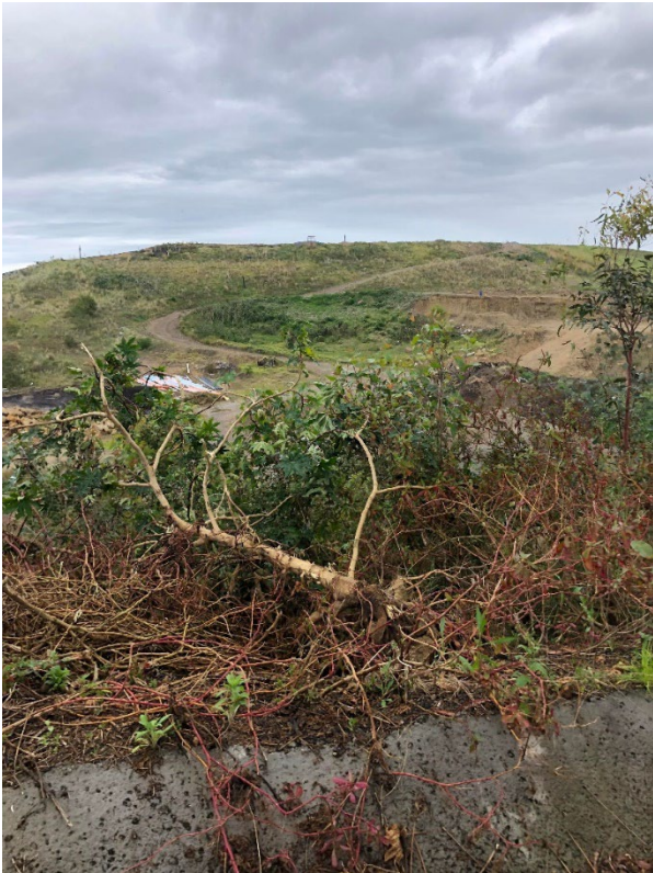
Photograph 7 – Weeds obstructing stormwater drains
