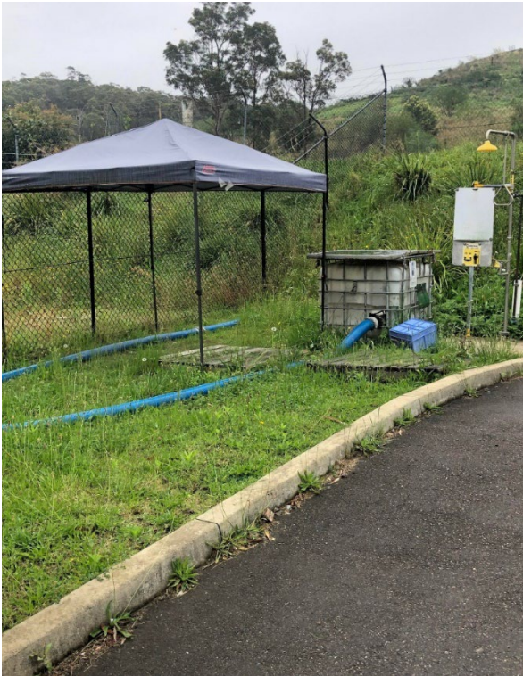
Photograph 3 – Temporary leachate loading station (unbunded on main access road)
