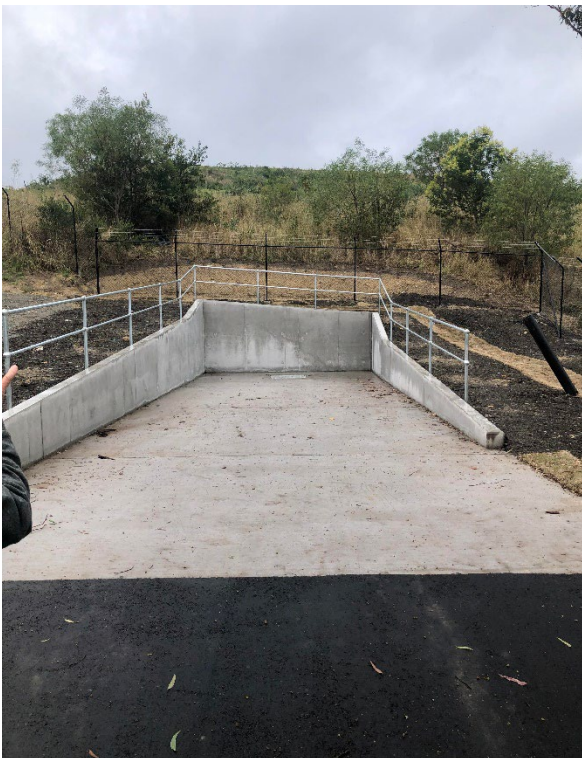
Photograph 2 – Construction area of a bunded area for leachate truck transfers
