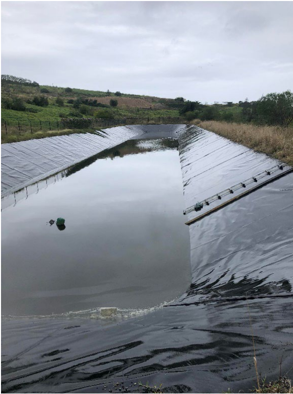
Photograph 5 – Overview of leachate pond 1
