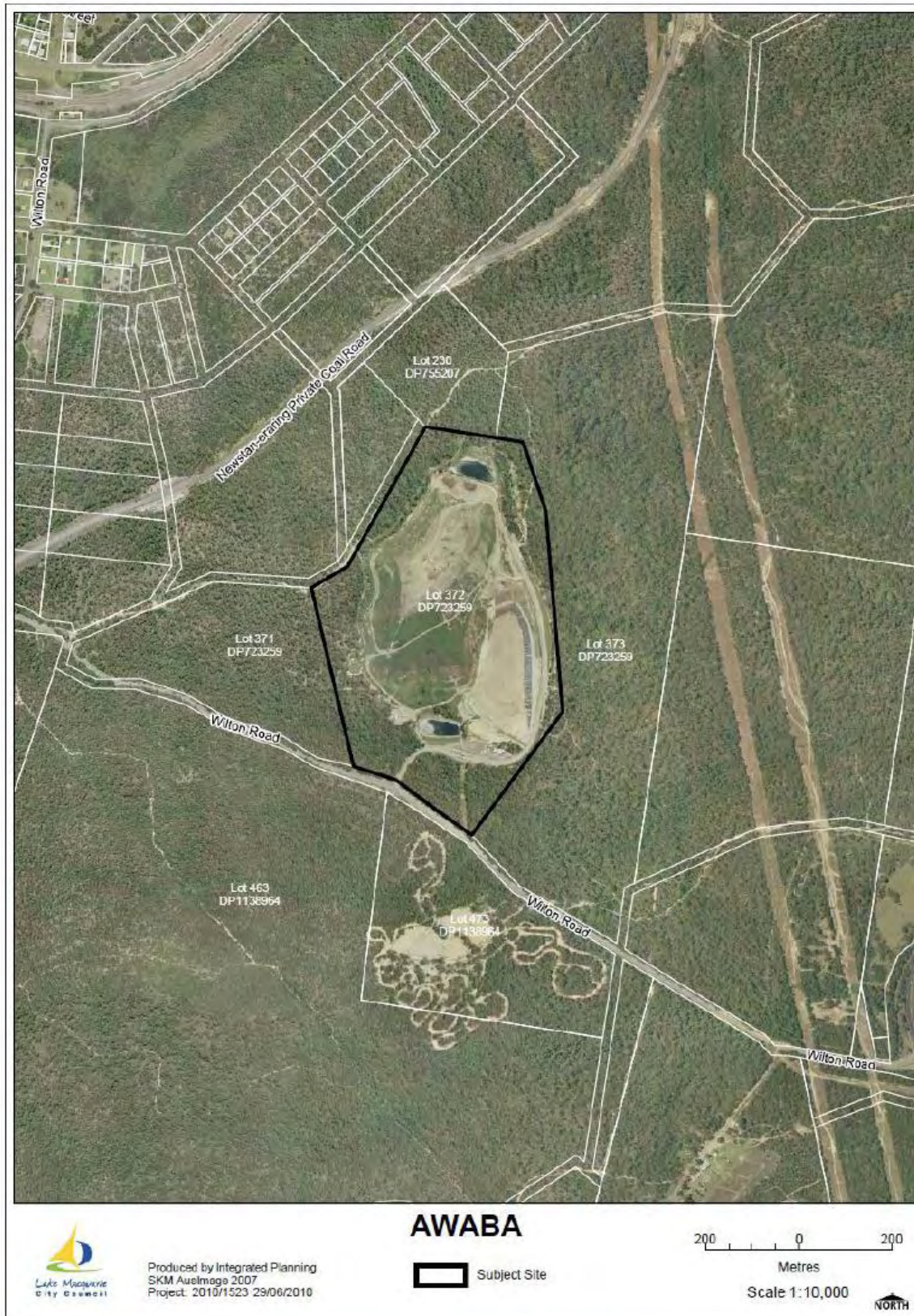
Figure 1 Location of Awaba Waste Treatment Facility
