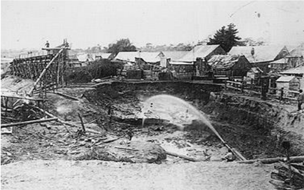
Figure 3: Water hoses were used to expose tin deposits (reproduced from Weidemann 1998)
