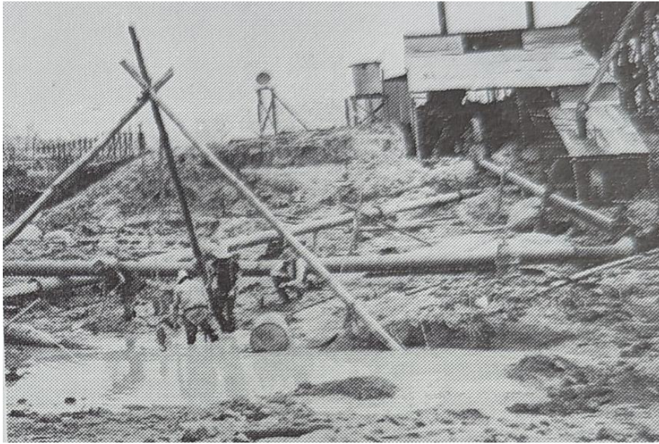
Figure 5: Tin mining caused significant disturbance (reproduced from Weidemann 1998)
