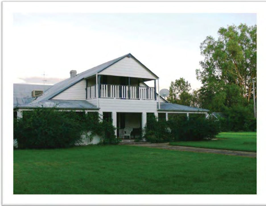
“Middle Creek South” House - Today
