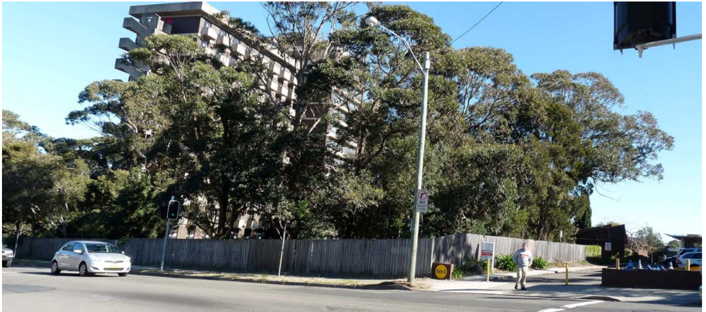
Figure 8 - View of site from Avoca Street (existing building to be demolished)
