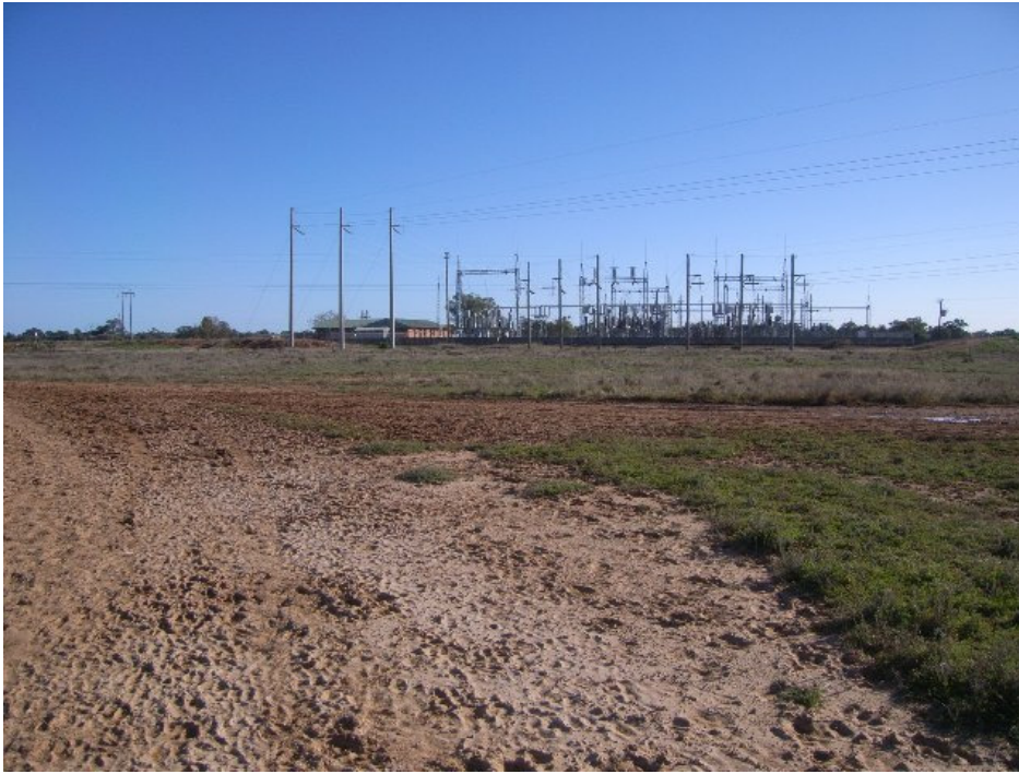
Plate 2 Looking north to existing substation.
