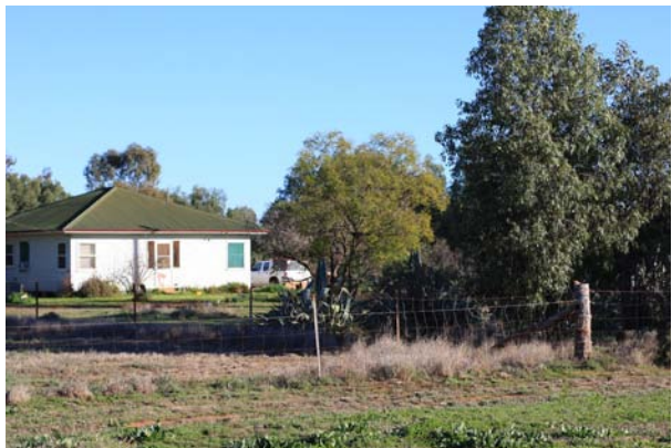
Rural residential housing along Hoskins Street.
