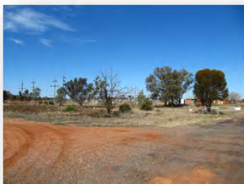
Photograph 29. Northern side of the sub-station with planted vegetation.
