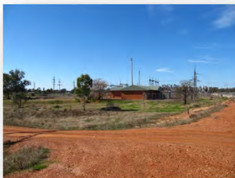
Photograph 28. Western side of sub-station.
