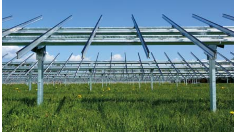
Example of a PV panel mounting structure (source: www.hpvm.com )
