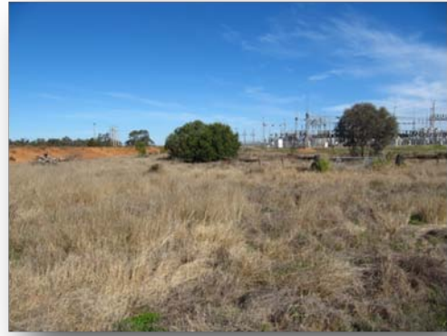
Photograph 30. Eastern side of sub-station.
