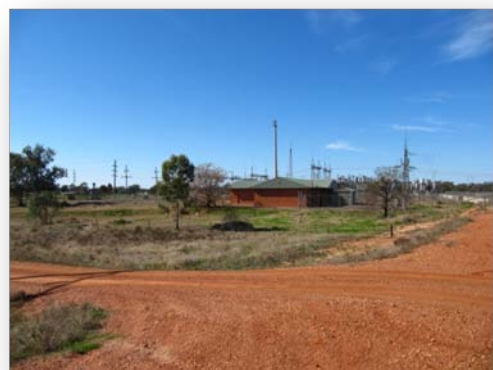
Photograph 28. Western side of sub-station.
