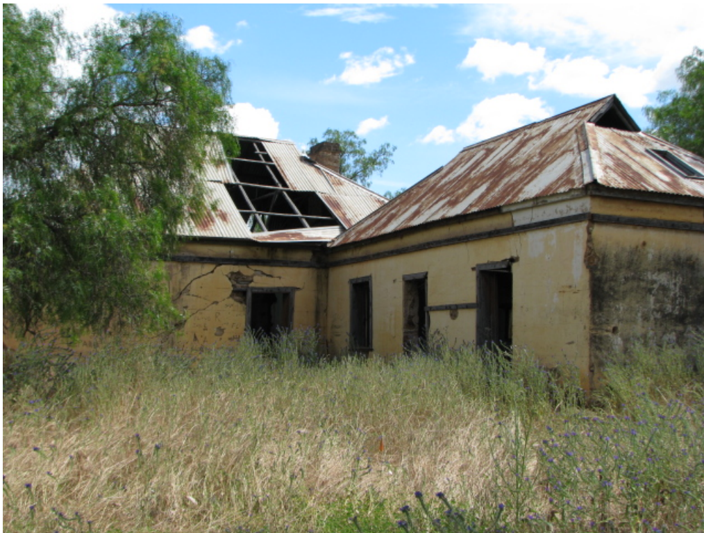
Figure 4.5. North east elevation that shows part of the roof in good condition and other sections loose and falling apart
