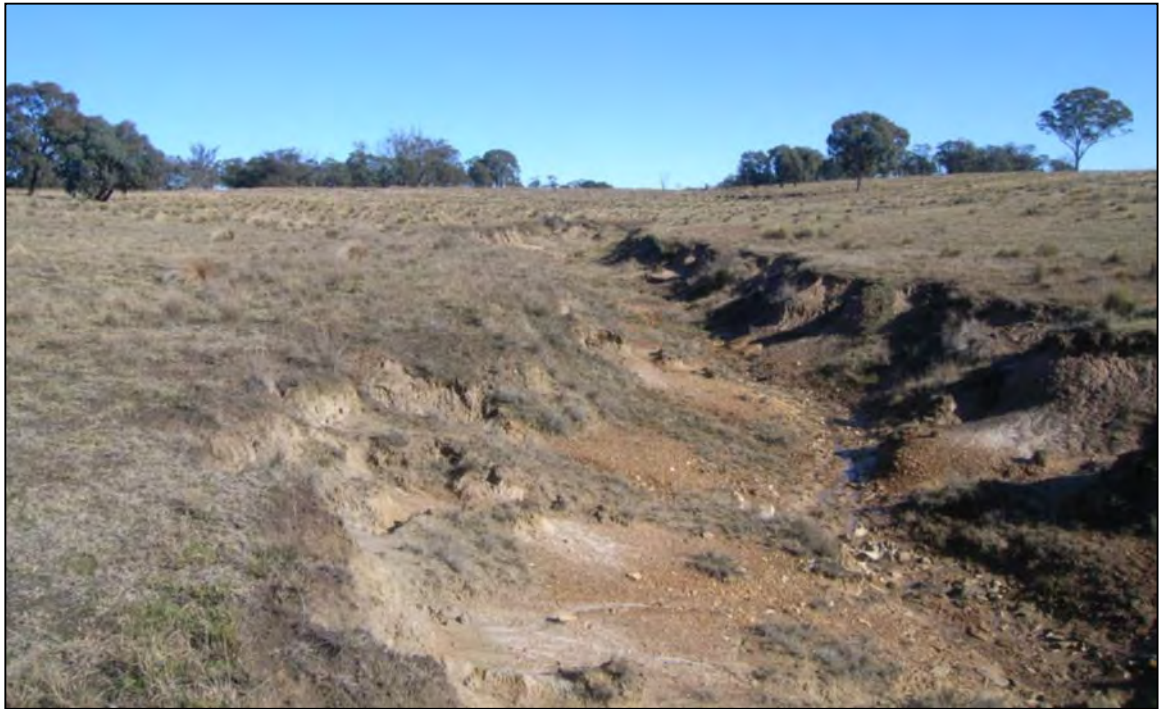
Plate 1. View of typical erosional scouring along drainage lines (tributary to Dry Creek), Survey Unit 8, looking west.
