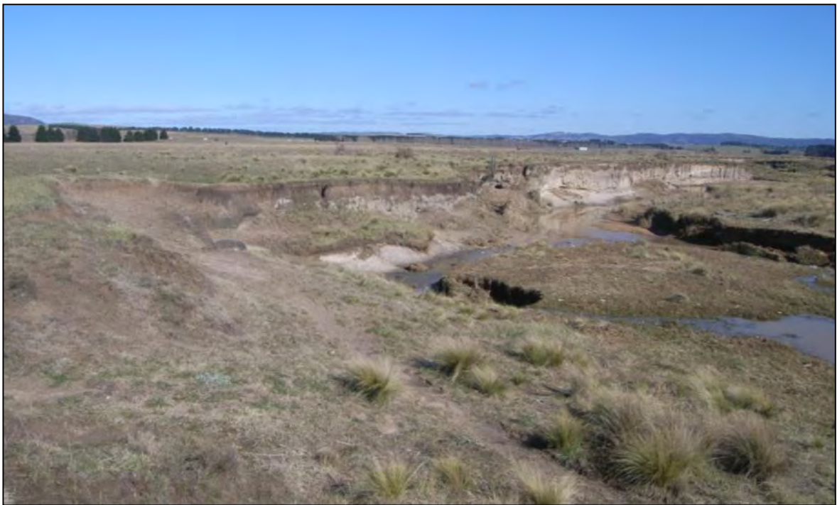
Plate 2. View of actively eroding creek bank (Bridge Creek), Survey Unit 30, looking southeast.
