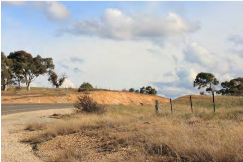
Embankments along Tarago Road.
