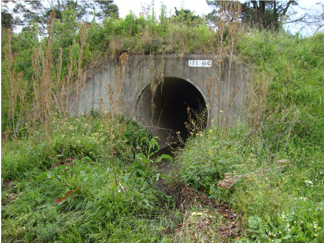
Photo 46b- Large pipe culvert in rail reserve on west side of Railway Street
