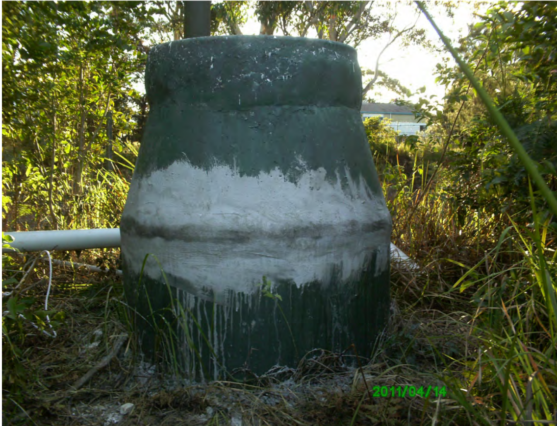
Photo 41-Sewer rising main manhole and vent pipe
