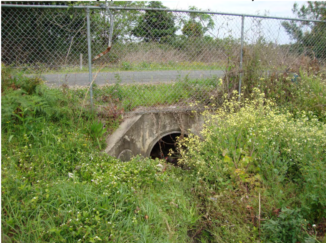
Photo 46c- Small headwall for pipe culvert under Railway Street, taking stormwater from large pipe culvert shown in previous photo.
