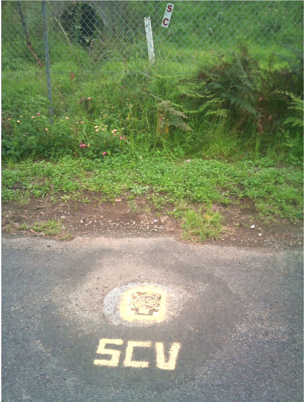
Photo 46a- Scour valve shown with Large pipe culvert in background leading into drainage system under Railway Street
