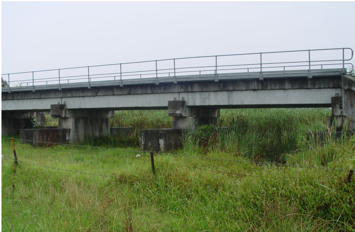
Figure 24: Railway Bridge #3 showing main flow path of Abernethys creek with waterway 3 flowing under one cell
