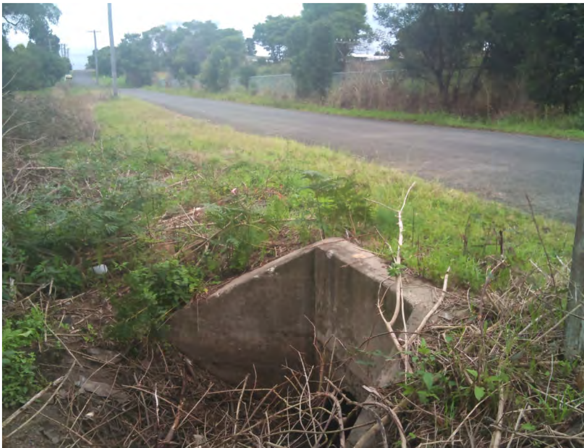
Photo 45- Stormwater headwall and culvert in Railway Street
