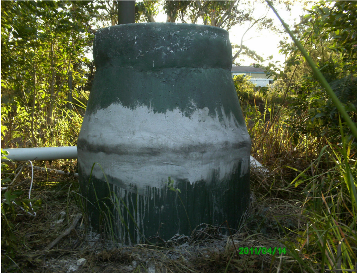
Photo 41-Sewer rising main manhole and vent pipe
