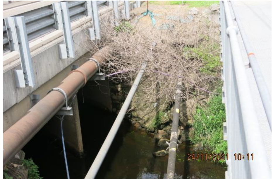
Photo 6: Example of existing services crossing Abernethy's Creek (24/11/2021)
