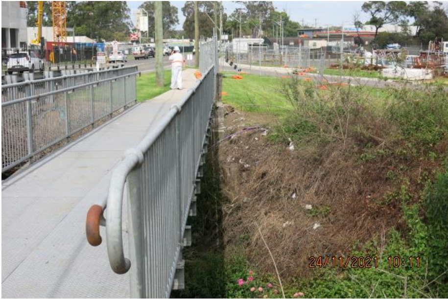
Photo 5: Looking south-west at the western bank of Abernethy's Creek in the vicinity of the proposed underbore (24/11/2021)
