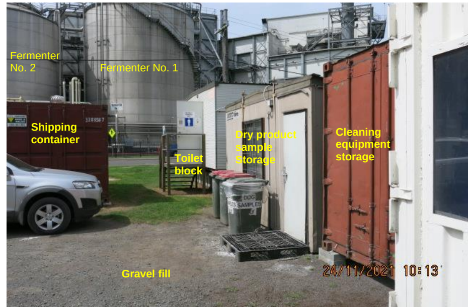
Photo 10: Looking south at Fermenter No's. 1 and 2 and approximate area where the proposed gas pipeline route is located. Note gravel fill, temporary buildings and shipping containers, which also occupy this area (24/11/2021)
