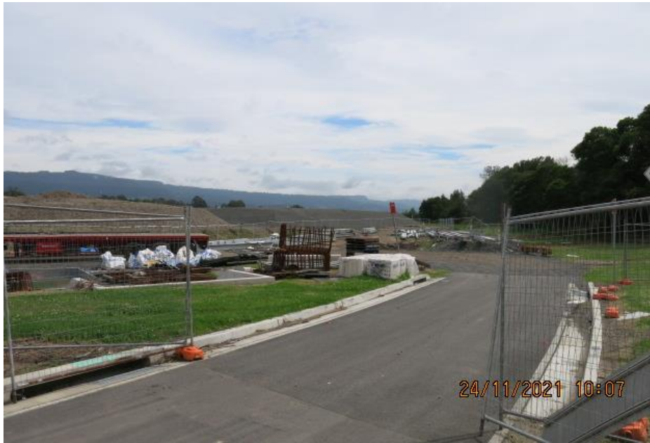
Photo 1: Looking north towards the packing plant development area at imported fill material (24/11/2021)
