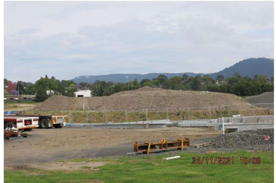
Photo 2: Brown-orange stockpile sourced from the Nowra Gaol construction site, classified as VENM (24/11/2021)
