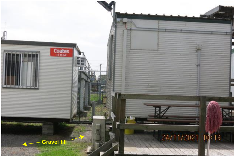
Photo 9: Looking east at the demountable buildings, noting gravel fill below and surrounding these structures (24/11/2021)
