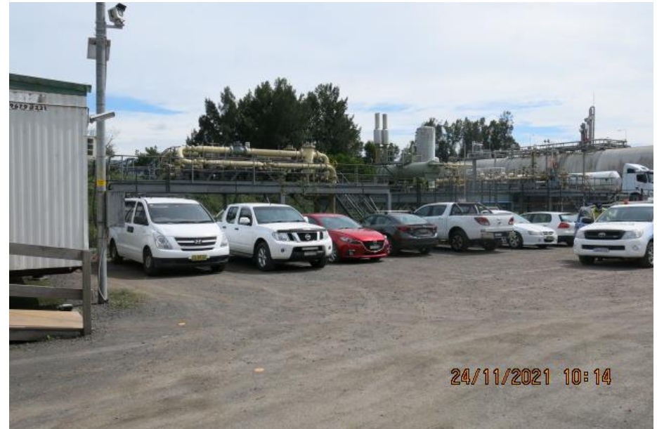
Photo 12: Looking north-east of the site at the existing gas facility located immediately north-east of the demountable buildings (24/11/2021)
