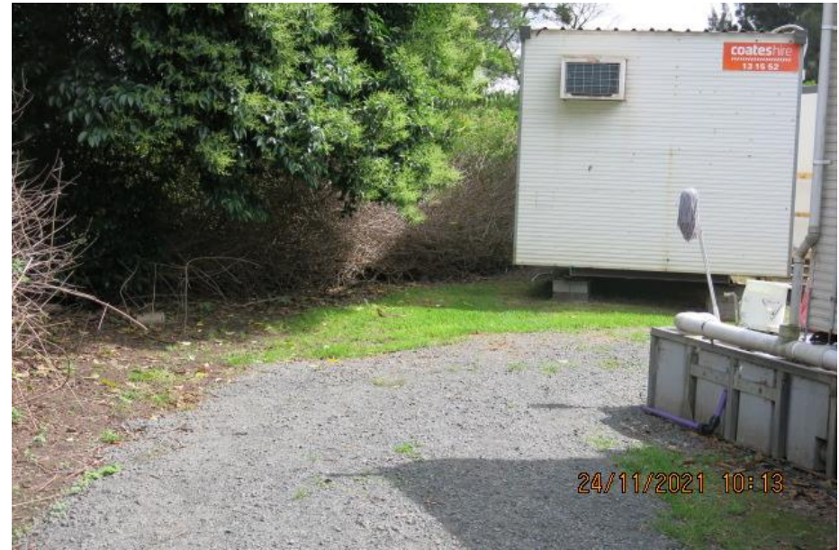
Photo 8: Area north of the site showing fill (grey gravel) imported as part of the temporary installation of demountable buildings and shipping containers (24/11/2021)
