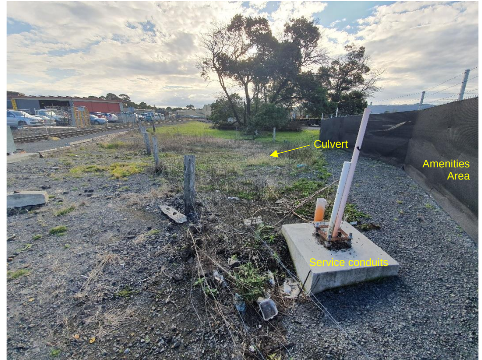
Photo 8: Looking north at the south-western corner of the site where fill material was observed. Note concrete culvert in background, refer to Photo 10 (17/6/2021).
