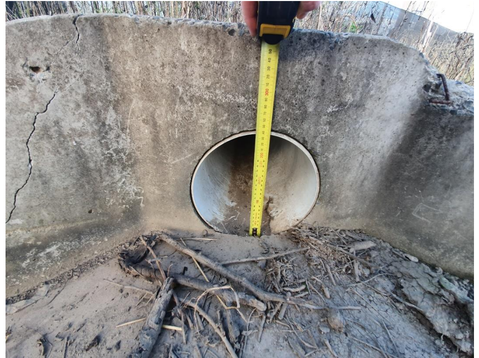
Photo 10: Looking at the concrete culvert within the south-western portion of the site (17/6/2021).
