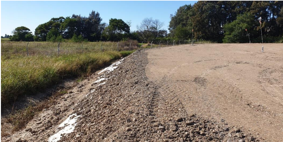
Photo 14: Looking east at the proposed gas pipeline route at the toe of the fill platform and adjacent thickly grassed area (23/4/2021).
