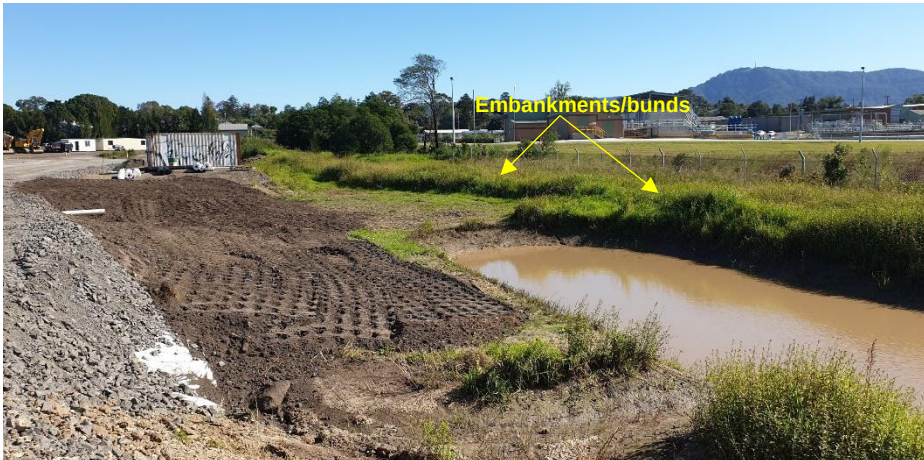
Photo 16: Looking north-west within the north-eastern portion of Lot 16. Note sediment pond on the right, and embankments and bunds in the background. The proposed gas pipeline will be located between the pond at the northern boundary of Lot 16 within grass area (23/4/2021).
