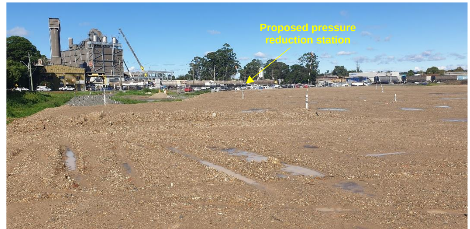
Photo 21: Looking south towards the section of proposed gas pipeline route that connects to the pressure reduction station (24/3/2021).
