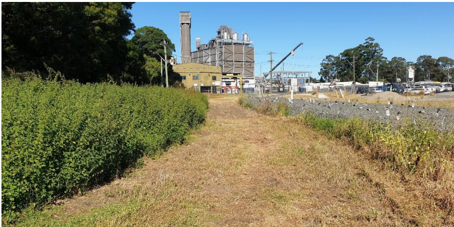
Photo 12: Looking south along the proposed gas pipeline route (23/4/2021).
