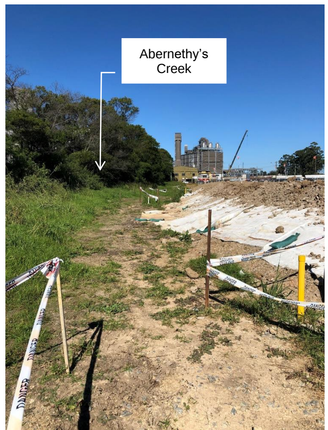
Photo 2: Looking south-east at the eastern section of the proposed gas pipeline alignment following a period of dry weather (23/4/2021).
