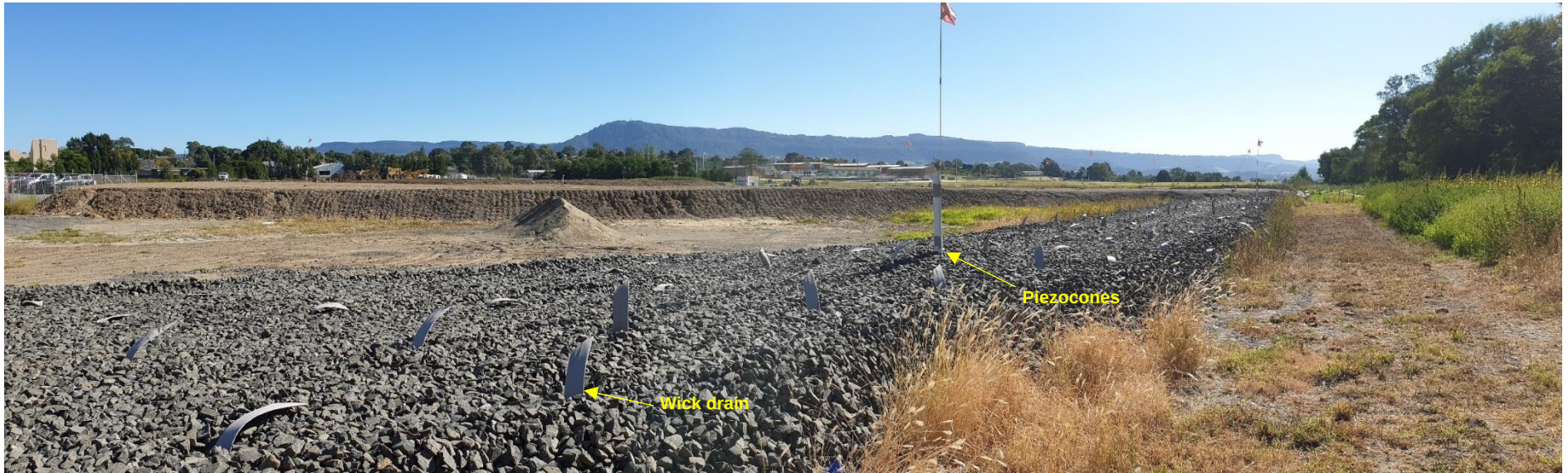
Photo 11: North-west at the latite gravel ramp in the foreground and weathered siltstone fill platform in the background. Note wick drains and piezocones installed within the latite gravel ramp (23/4/2021).
