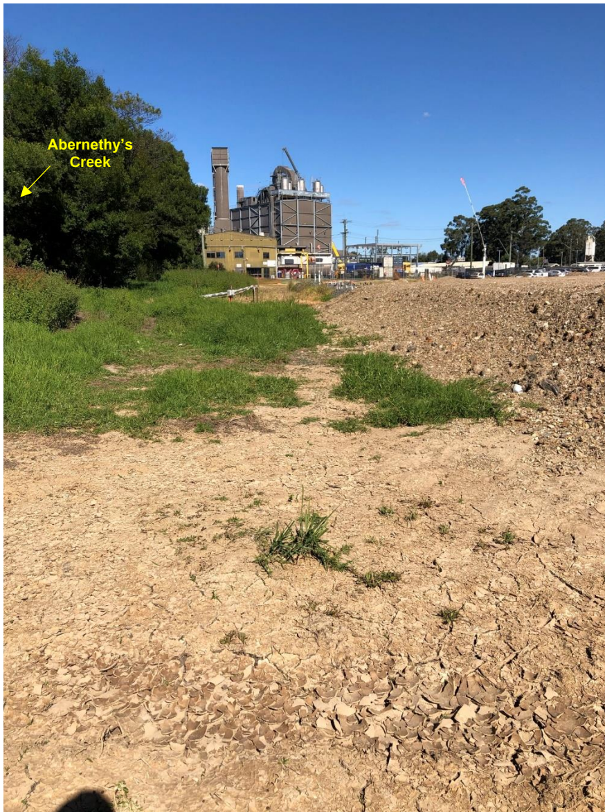
Photo 20: Looking south along the proposed gas pipeline route, located between the toe of the fill platform and Abernethy's Creek (23/4/2021).
