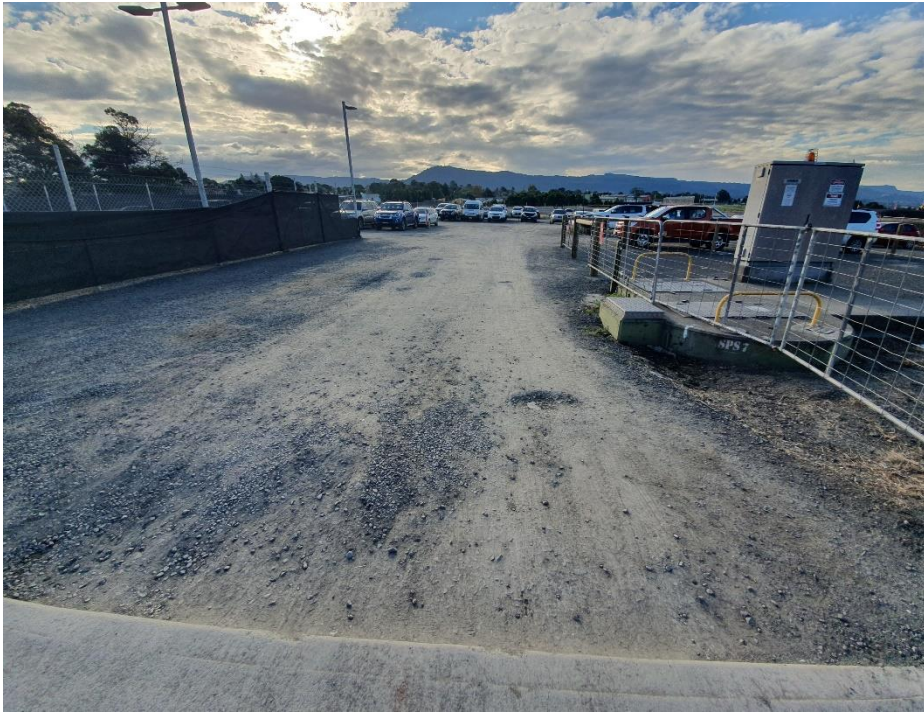
Photo 5: Looking north along the access driveway to the carparking area the occupies the northern one third of the site. Note sewer pumping station in the right-hand side of photo (17/6/2021).
