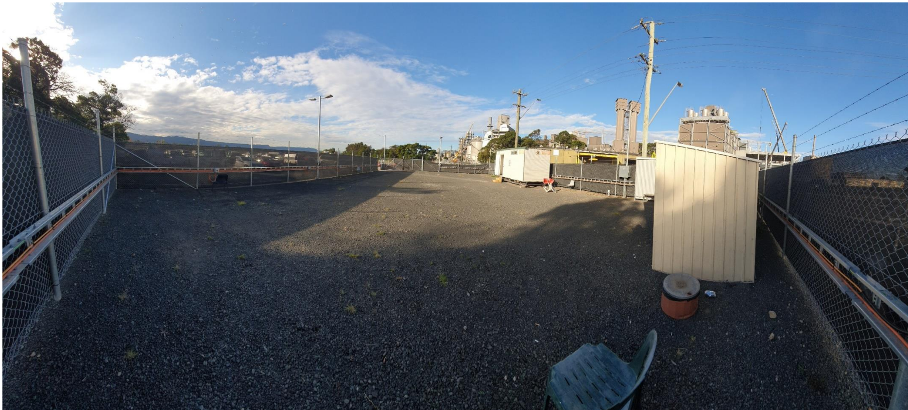
Photo 4: North-east at the southern two-thirds of the site at the amenities area (17/6/2021).
