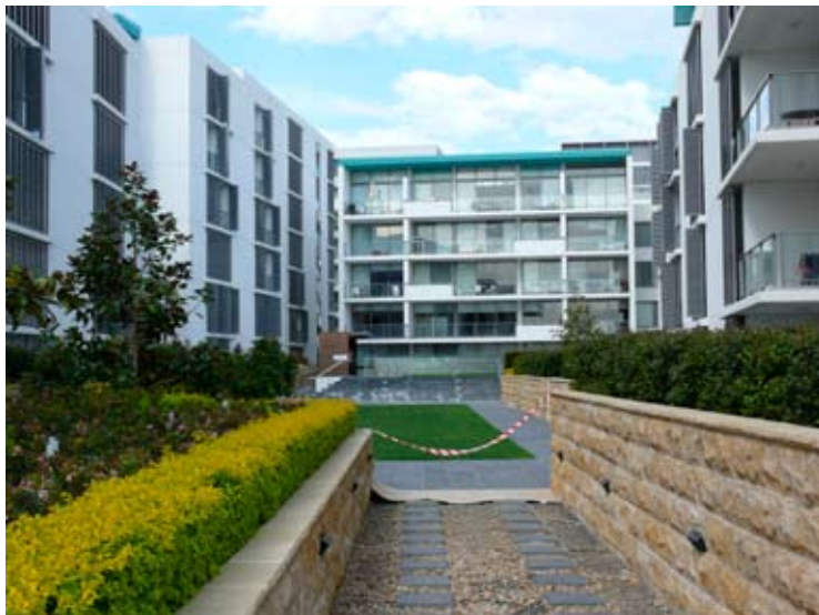
Courtyard apartment housing within internal private spaces
