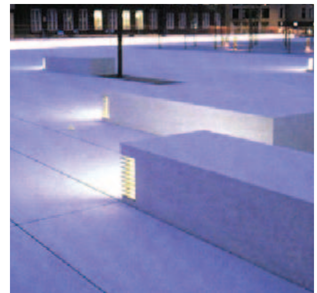
Suspended precast concrete unit deck with opportunities to integrate lighting and signage
