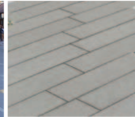
Type 4: Lookout : Precast concrete units
