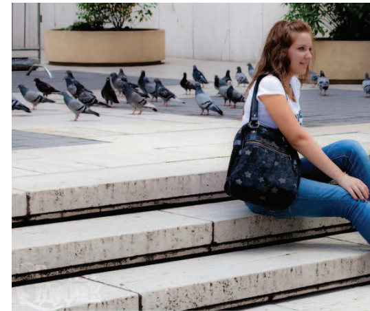
Step Type 2: Seat/ access steps 600 mm wide x 155 mm high treads precast concrete
