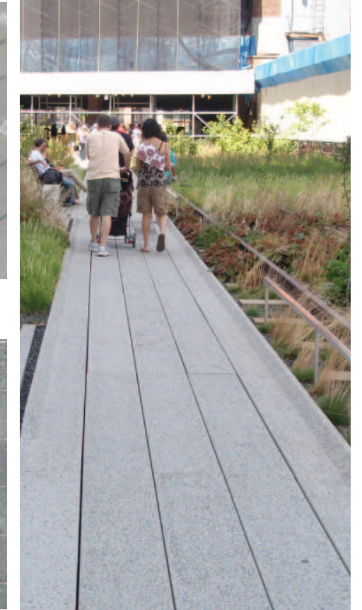
Type 4: Lookout : example of Precast concrete units Highline project, New York
