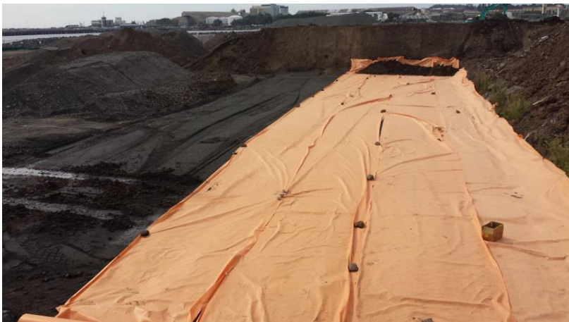
Figure 4-4 Encapsulated asbestos impacted stockpile. Photograph shows orange geo fabric encapsulating layer placed directly above the contaminated soils
