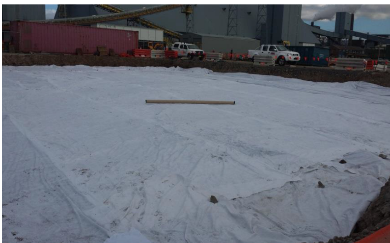
Figure 4-5 Encapsulated asbestos impacted stockpile with centre point at 307405.8862E, 6183655.792N. Photograph shows white geo fabric encapsulating layer placed directly above the contaminated soils.
