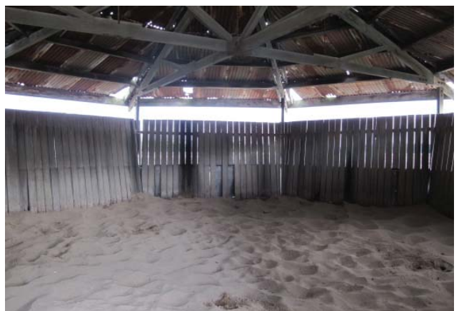
Figure 3.13 Interior of the Southern Sand Roll
