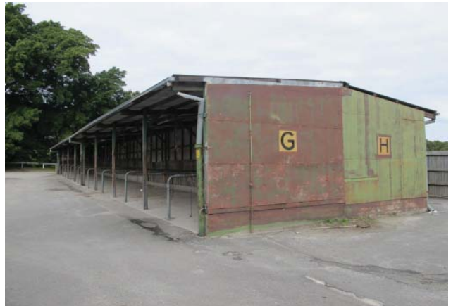
Figure 3.11 Shows Stripping Stalls G and H, looking to the east
