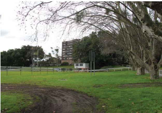
Figure 3.16 View to the track crossing showing the Stewards' Tower and Office
