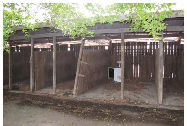
Figure 3.7 East side of Stripping Stall C
