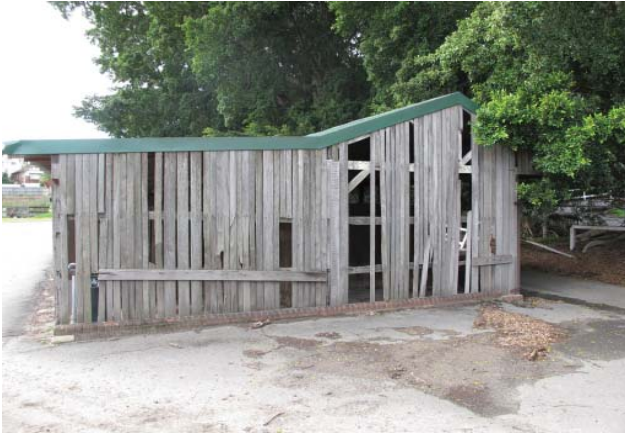
Figure 3.8 Southern end of Stripping Stall C
