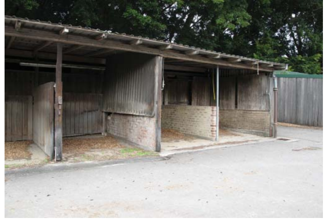
Figure 3.9 Stripping Stalls D
