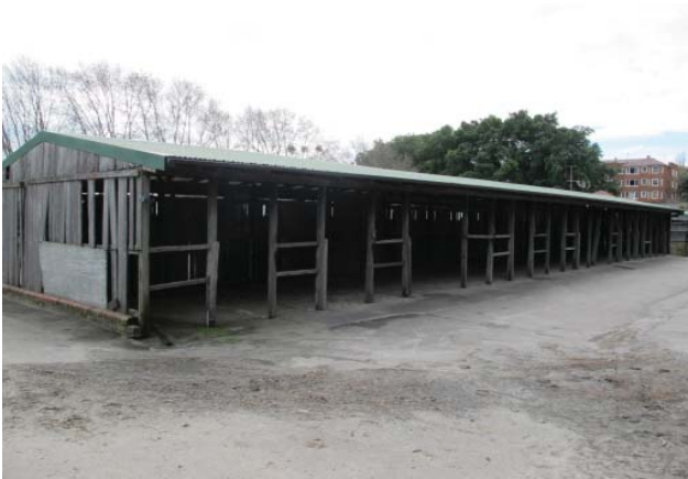
Figure 3.10 South and East elevation of Stripping Stall E
