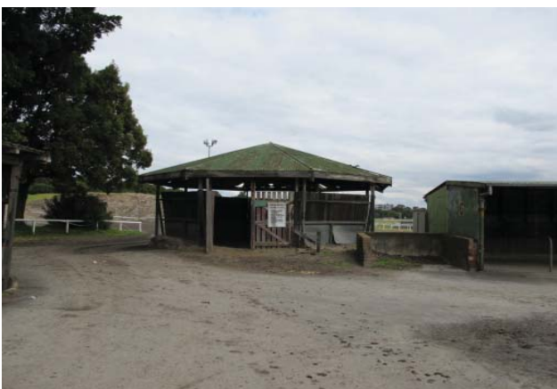
Figure 3.12 Southern Sand Roll, adjacent to Stripping Stalls G and H
