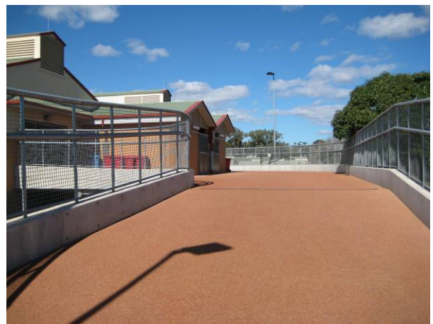
Picture 6 – Ramp for horse access to first floor stables, which is also wide enough to accommodate vehicles if required.
