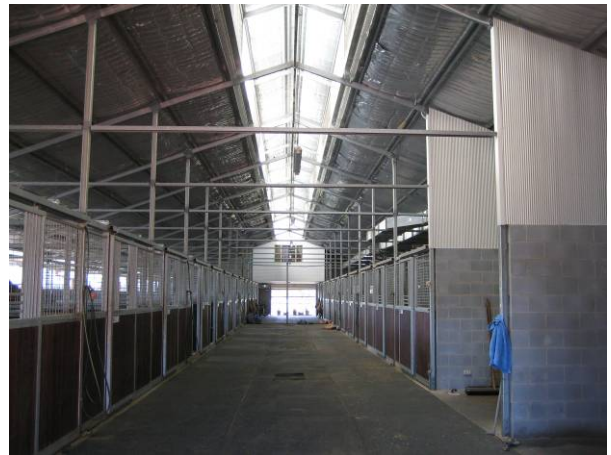
Picture 4 – Internal layout of first floor stables with large side windows and a large skylight to provide natural sunlight and ventilation.
