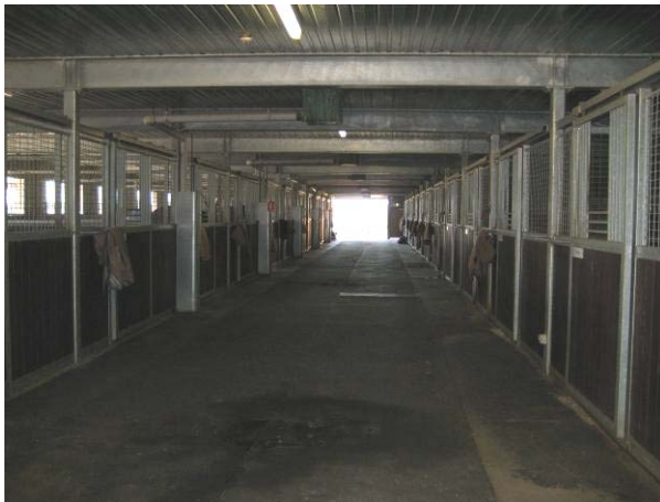
Picture 3 – Internal layout of ground floor stables with large windows along sides to provide for natural sunlight and ventilation.
