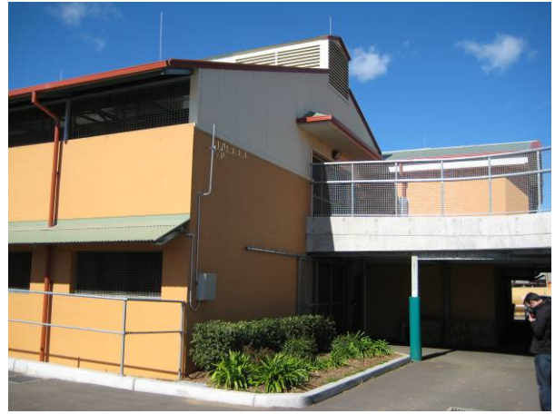
Picture 2 – Dual entry to Stable facility, with elevated ramp access to first floor stables.
