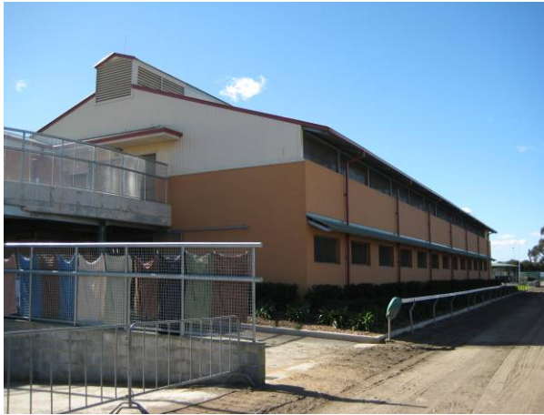
Picture 1 – External appearance of two-storey Stable Building
