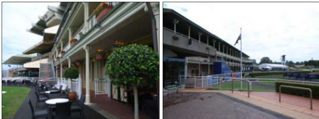
Figure 11: The front area of the Officials Stand, at left and the fenced off judging area at right.
