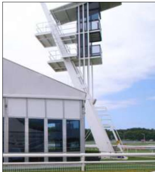
Figure 39: The 2004 constructed Stewards Tower is adjacent to the Officials Stand and to this temporary grandstand.
