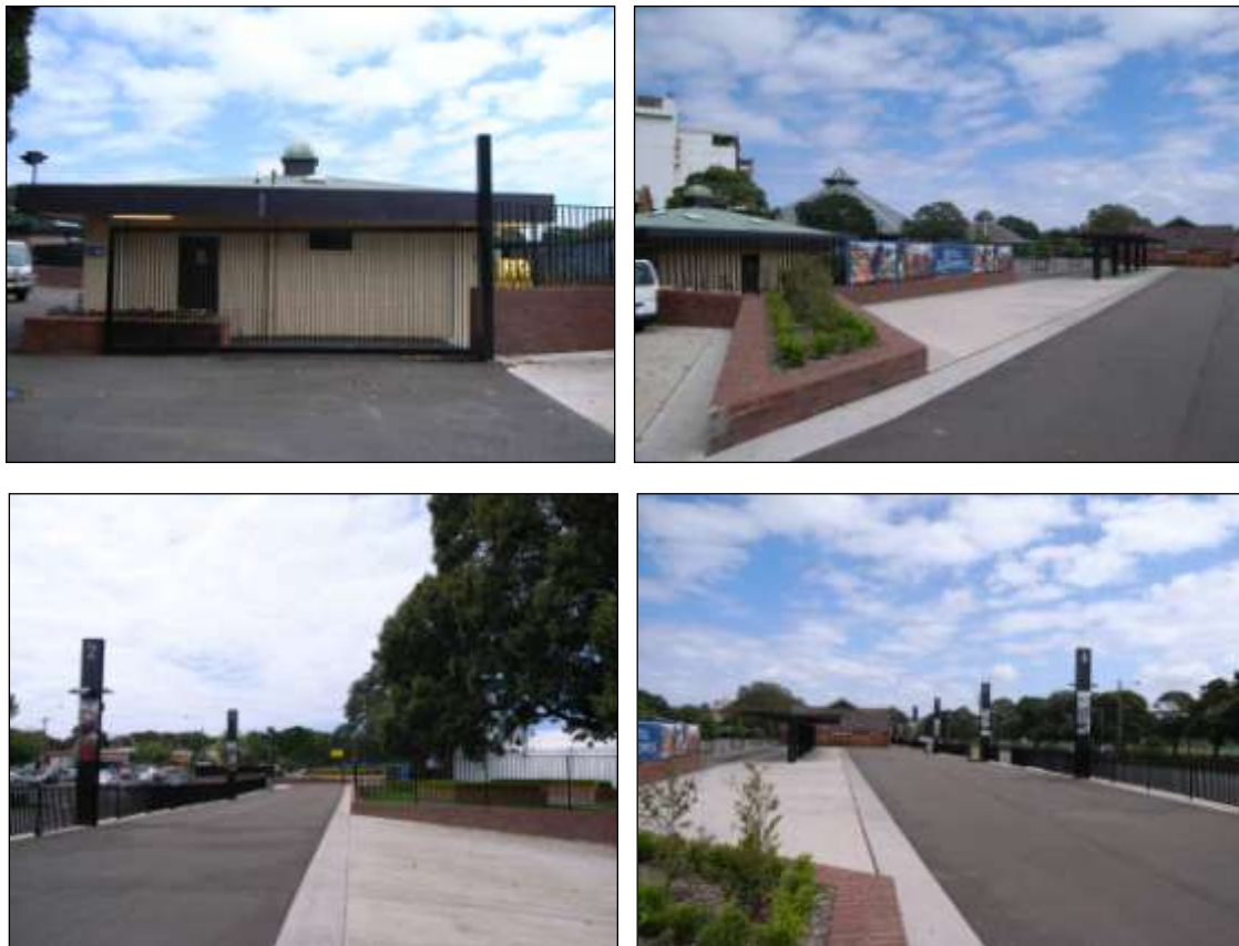
Figure 14: Views of the Alison Road section of the Spectator Precinct and its buildings and the extended bus parking area
