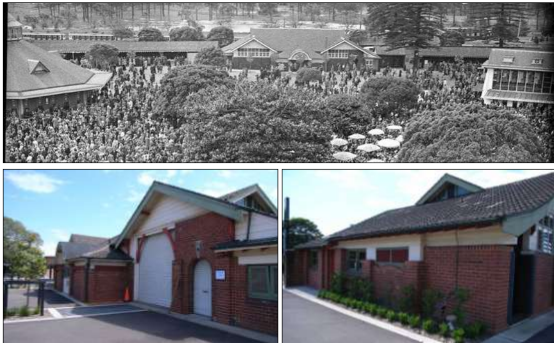
Figure 38: Views of the Swab Building, former men's lavatory. Top, the view in 1937 with the October Derby Day crowds. Above, the view in October, 2011 during the site visit.
