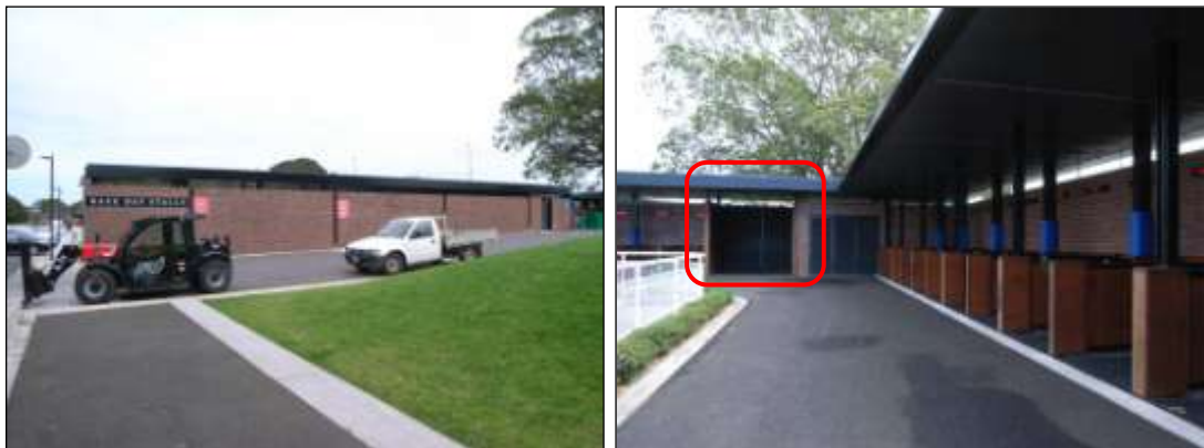
Figure 9: External and internal views of the Race Day Stalls. The area indicated at right is proposed for underground access tunnel as part of current or future works.
