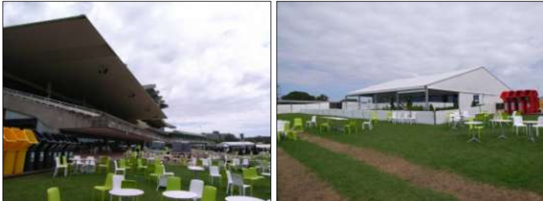
Figure 10: View in front of the grandstands; left, in front of the Paddock Stand, with the QE II and Officials Stands and a temporary stand in the background. Right, the temporary grandstand located south of the Paddock Stand.
