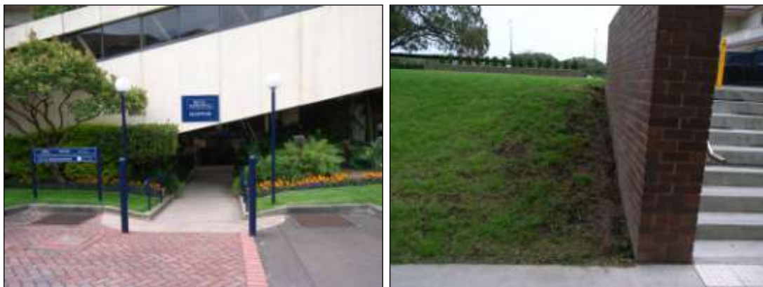
Figure 8: Left, the entry to the lower level and front race track lawn of the Paddock Stand. Right, the raised lawn area in between the back of the Teahouse and the existing Race Day Stall. Formerly, this was a roadway and the St Leger area entry turnstiles
