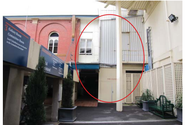
Figure 7.5 Shows the existing poorly resolved junction at the rear of the Queen Elizabeth II Stand and the Official Stand
