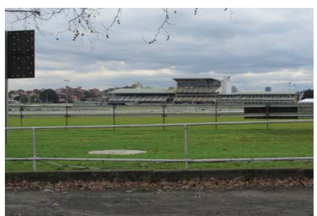
Figure 7.7 View to the existing stands from the other side of the Racecourse showing the existing relationship between the Queen Elizabeth II
