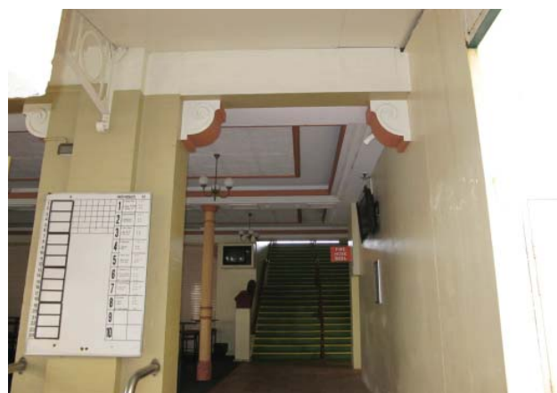
Figure 7.4 Interior wall of the junction between the Official Stand and the Queen Elizabeth II Stand
