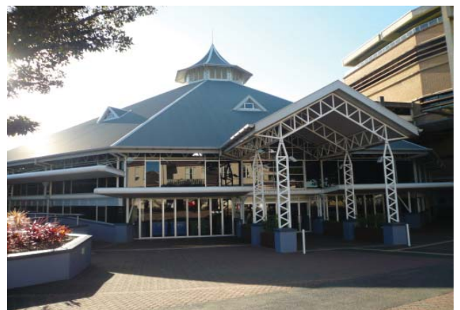
Figure 3.13 The Randwick Pavilion extension to the Totalisator Building that is to be demolished as part of the proposed development
