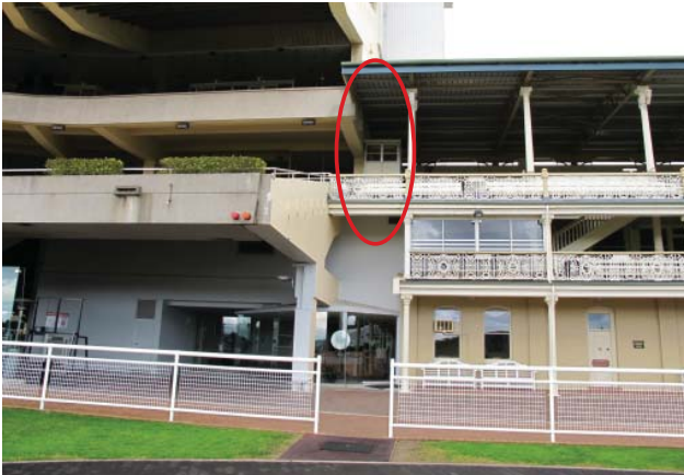
Figure 7.2 Shows the existing poorly resolved junction between the Queen Elizabeth II Stand and the Official Stand
