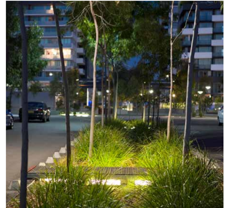
Garden beds and tree pits also benefit from passive irrigation
