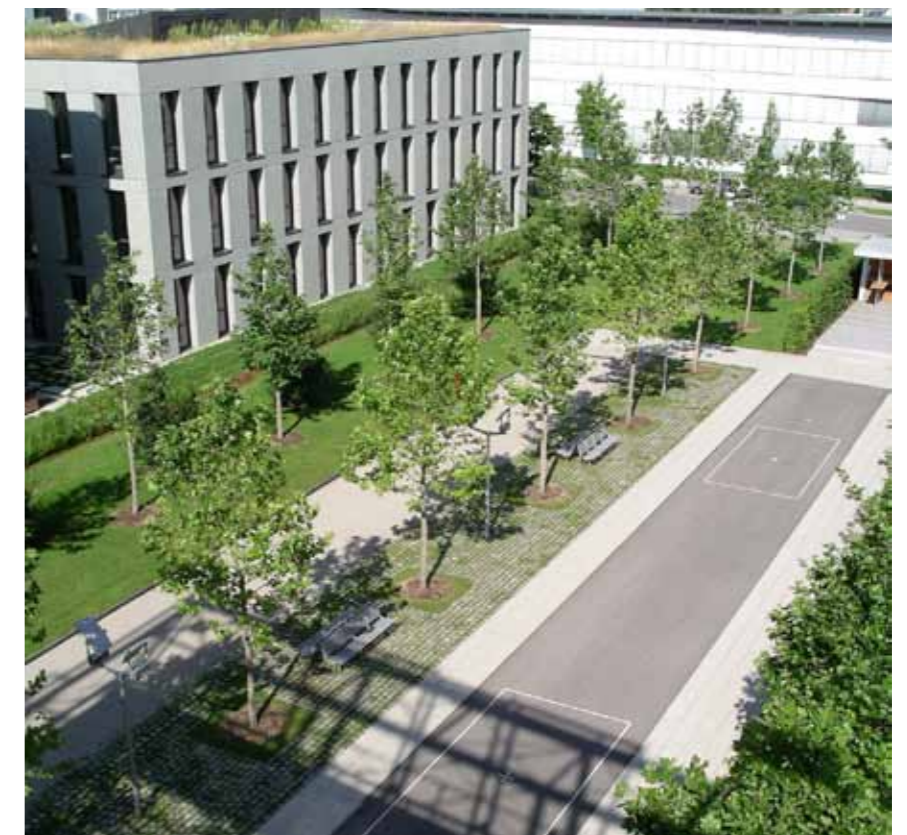
Insitu concrete headers frame paving
