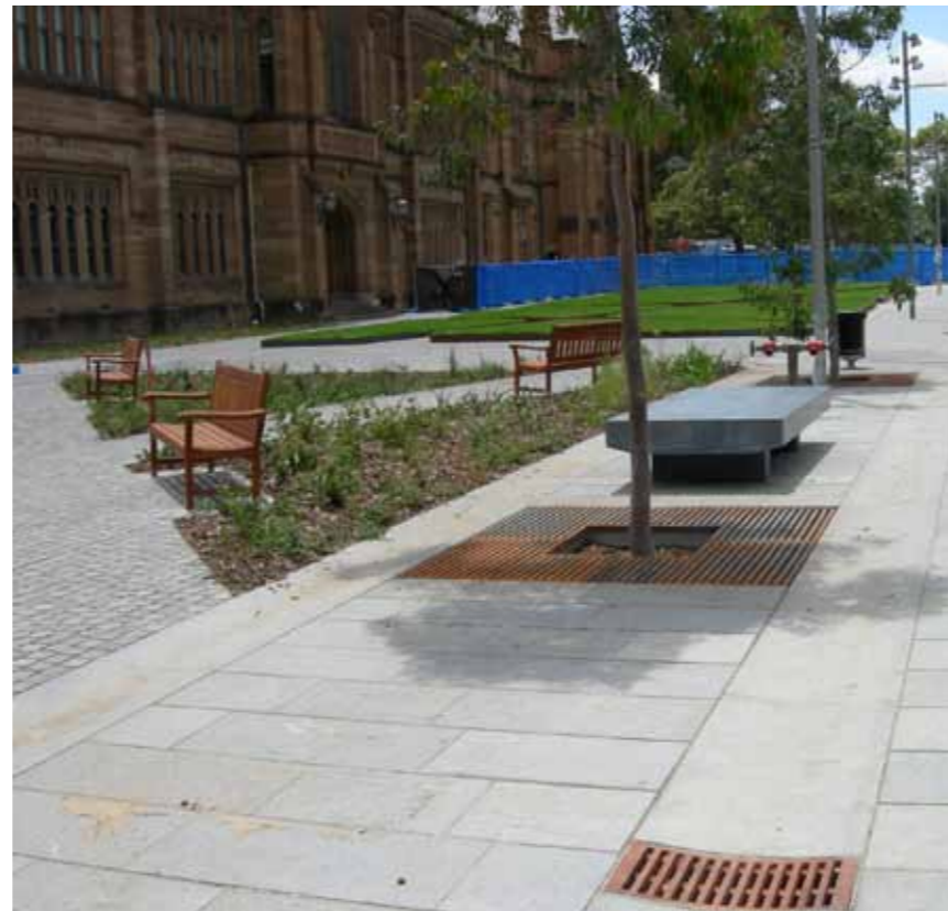
Drainage grates and other service pits are intergrtaed into the paving layout
