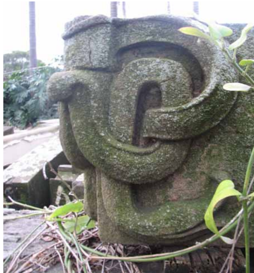
Existing sandstone relics are intergrated into the spectator precinct
