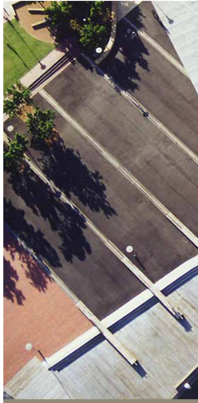
Structure to the ground plane emphasises the architectural setout
