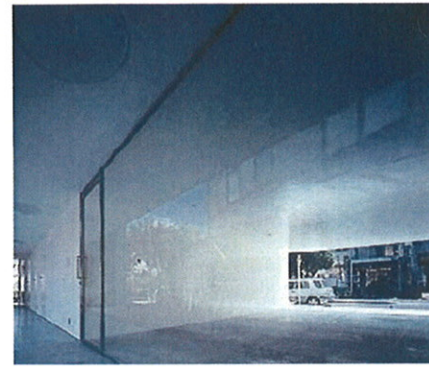
WINDOWS - TRANSPARENT GLAZED PANEL & POWDERCOATED ALUMINIUM FRAME (DARK COLOUR) (W)
