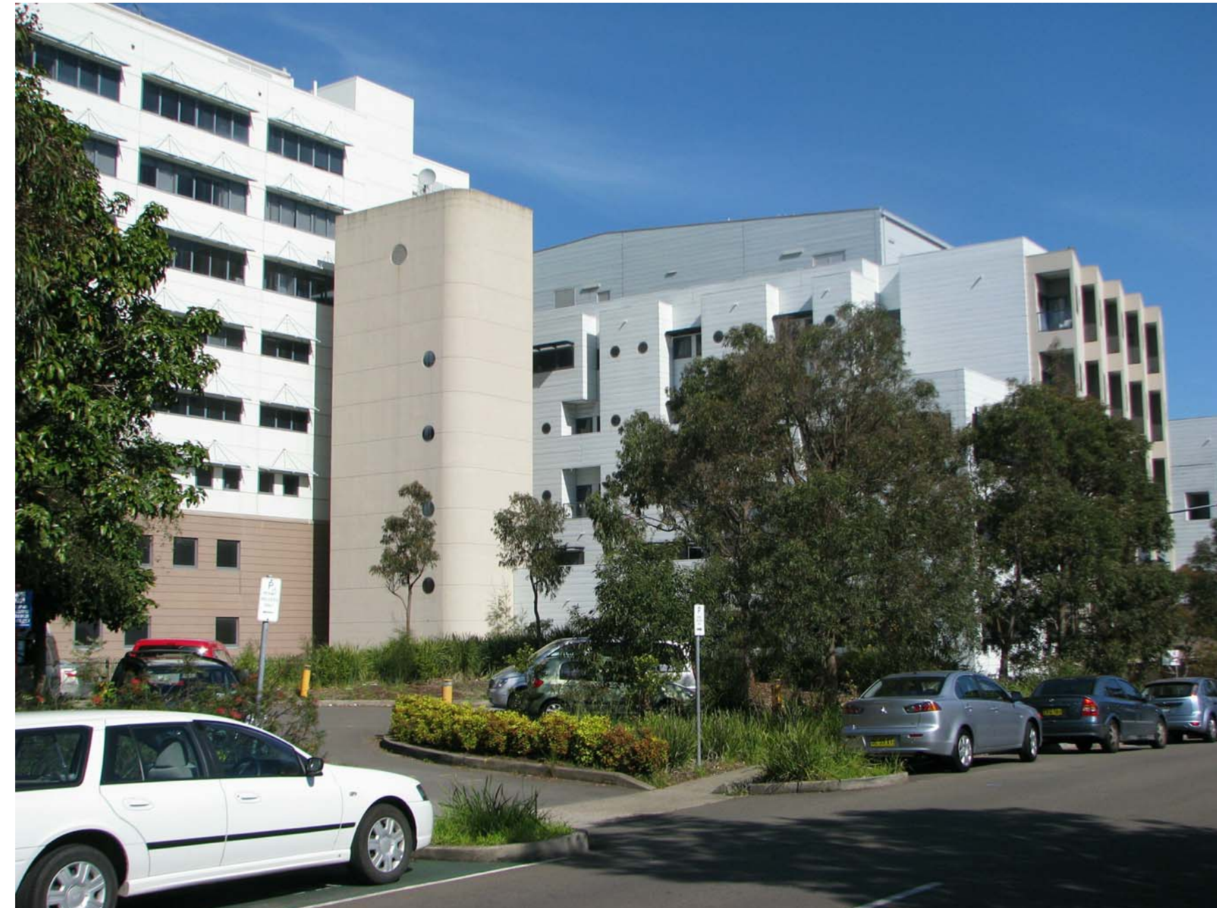
3 VIEW LOOKING EAST FROM HOSPITAL ROAD
